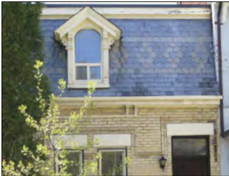
Surviving polychromatic slates and roof dormer on this Second Empire Roof give guidance for re-instating lost detail on adjacent houses should opportunity arise.
