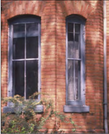
Restored wooden storm window (Cabbagetown example)
