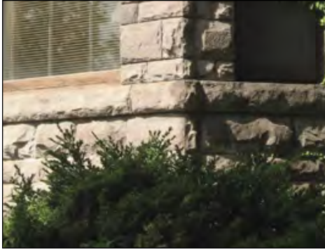
Rusticated sandstone foundation/ground floor typical of Annex Style houses, and later Romanesque style “Bay-n-Gable” houses
