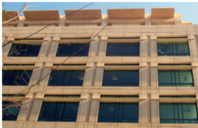
Figure 2: A "sustainable" façade design, including operable windows for natural ventilation and fenestration to shade high-performance glazing.
