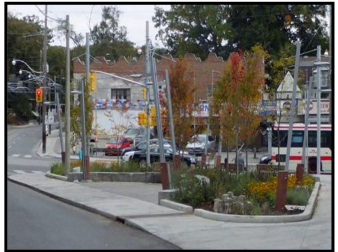
Green Infrastructure Example: Bioretention for street corners
