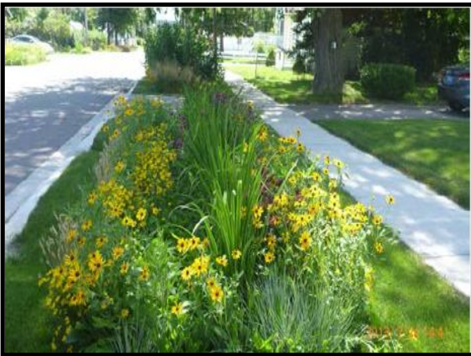
Green Infrastructure Example: Bioswales for ditched roads
