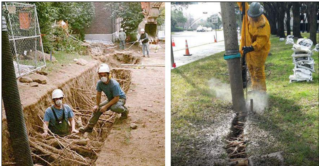
Figure 10.3.22 – Pneumatic (left, photo: djc.com) and hydraulic (right, photo: Ruskins.co.uk) excavation techniques minimize damage to tree roots.
