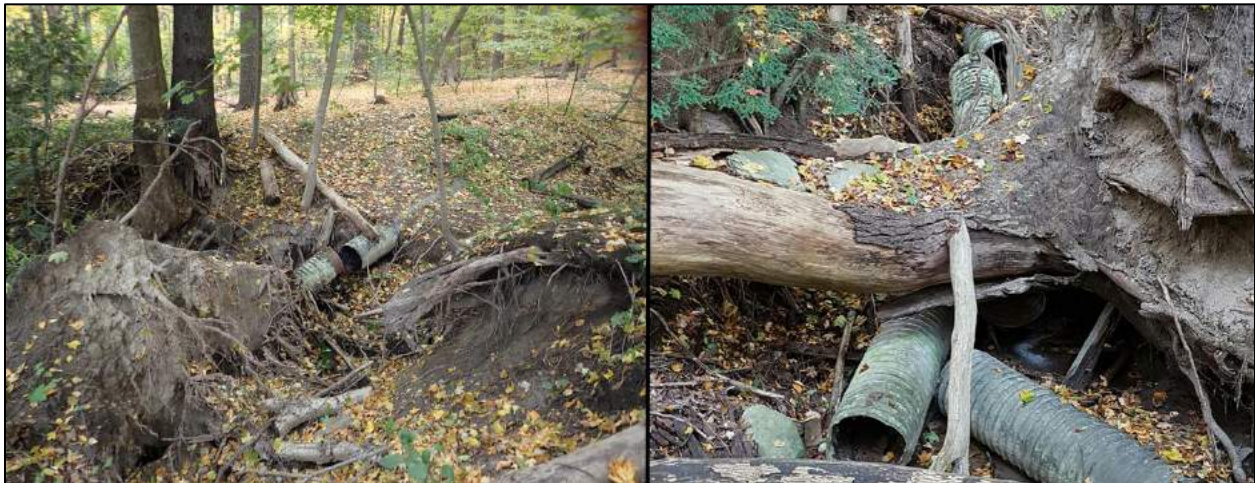
Figure 10.3.24 – Undermined Sewer Pipe Causing Erosion at Site 1
