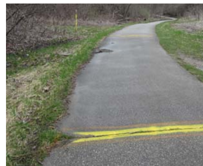
Cracking / broken asphalt
