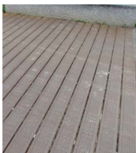
Weathering steel decking
