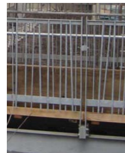
Evergreen Brick Works - galvanized steel railing
