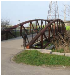
Truss bridge with railings
