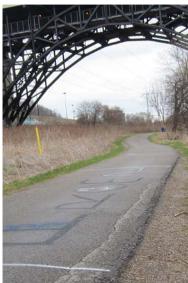
Broken asphalt edges of trail
