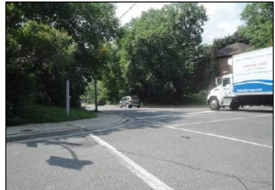
Figure 6-4 Sightline at St. Leonard's Ave. to NB Vehicle on Mount Pleasant Ave.
