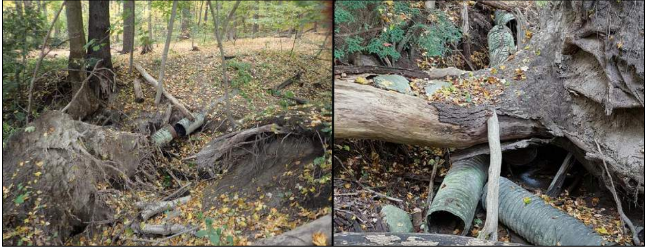
Figure 3.1: Undermined Sewer Pipe causing Erosion at Site 1
