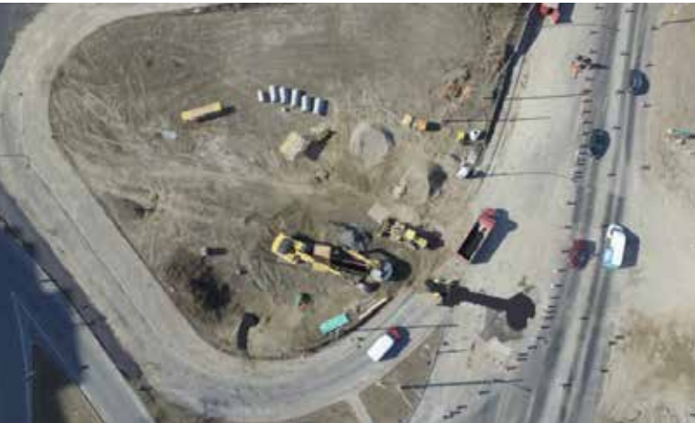
Underground utilities are being installed crossing Kipling Avenue for new watermains, storm and sanitary sewers.
