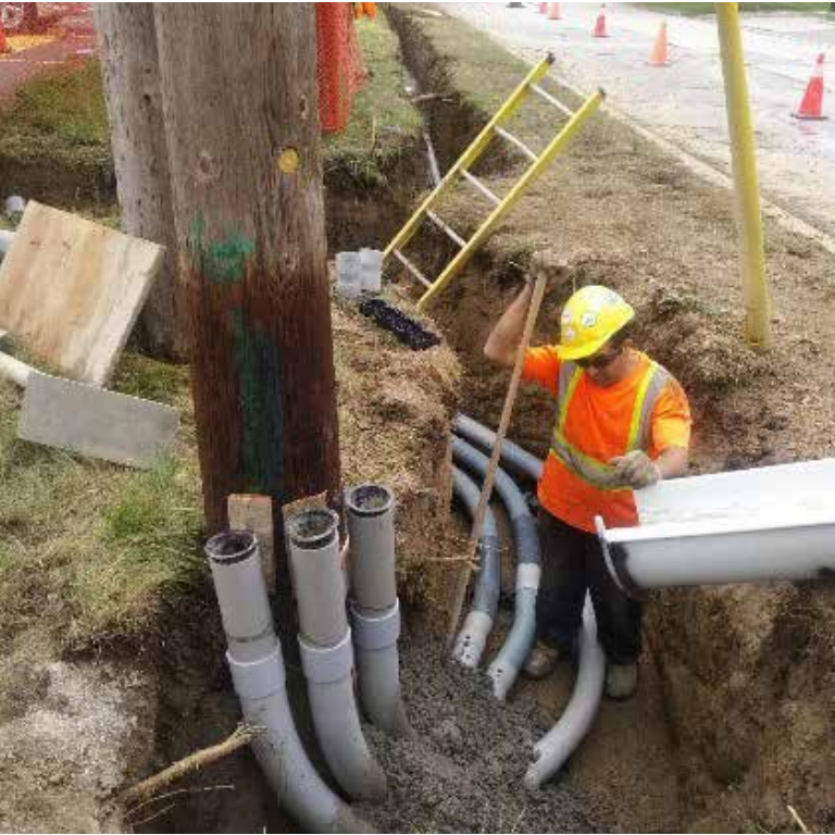
An underground Hydro duct bank has been constructed on Dundas between Auckland Road, to Jopling Avenue.
