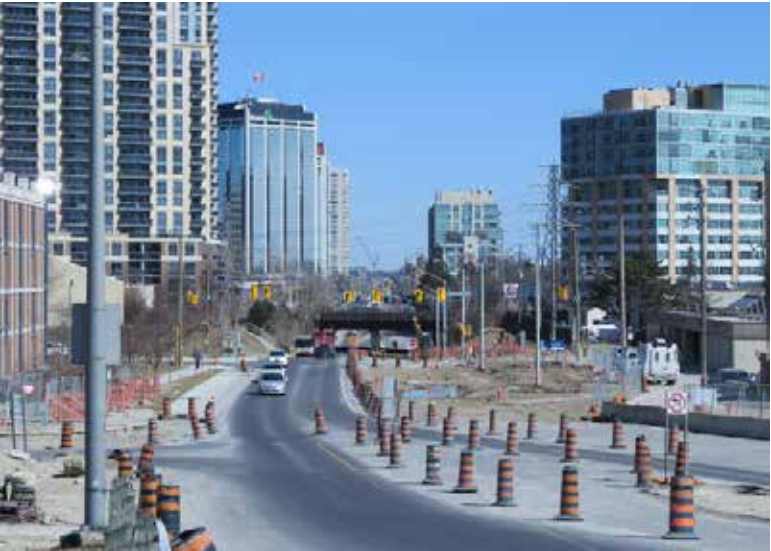
Along Bloor Street West, crews are installing temporary asphalt, new watermains, separate storm and sanitary water sewers, and streetscaping (including landscaping, street lighting and underground utilities).
