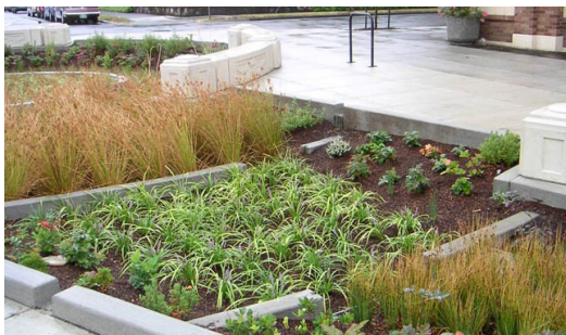
Figure 9.13: Bioswale Example
