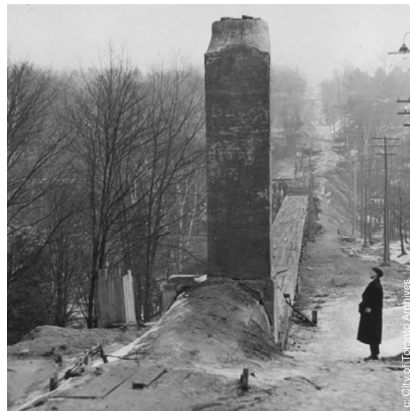
Considerable modifications have occurred over the years. This image is of the sewer system being constructed along Bloor Street West in the early 20th century.
