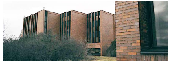
Existing at 1150 Eglinton Ave E
