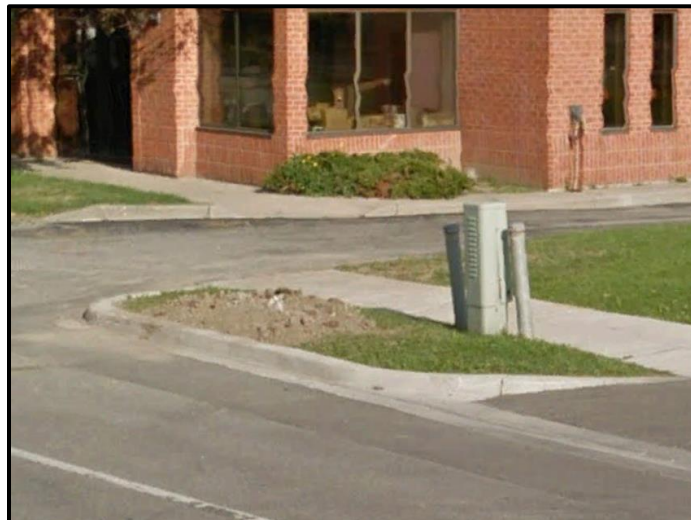
Figure 4-12 Telecommunication Pedestal
