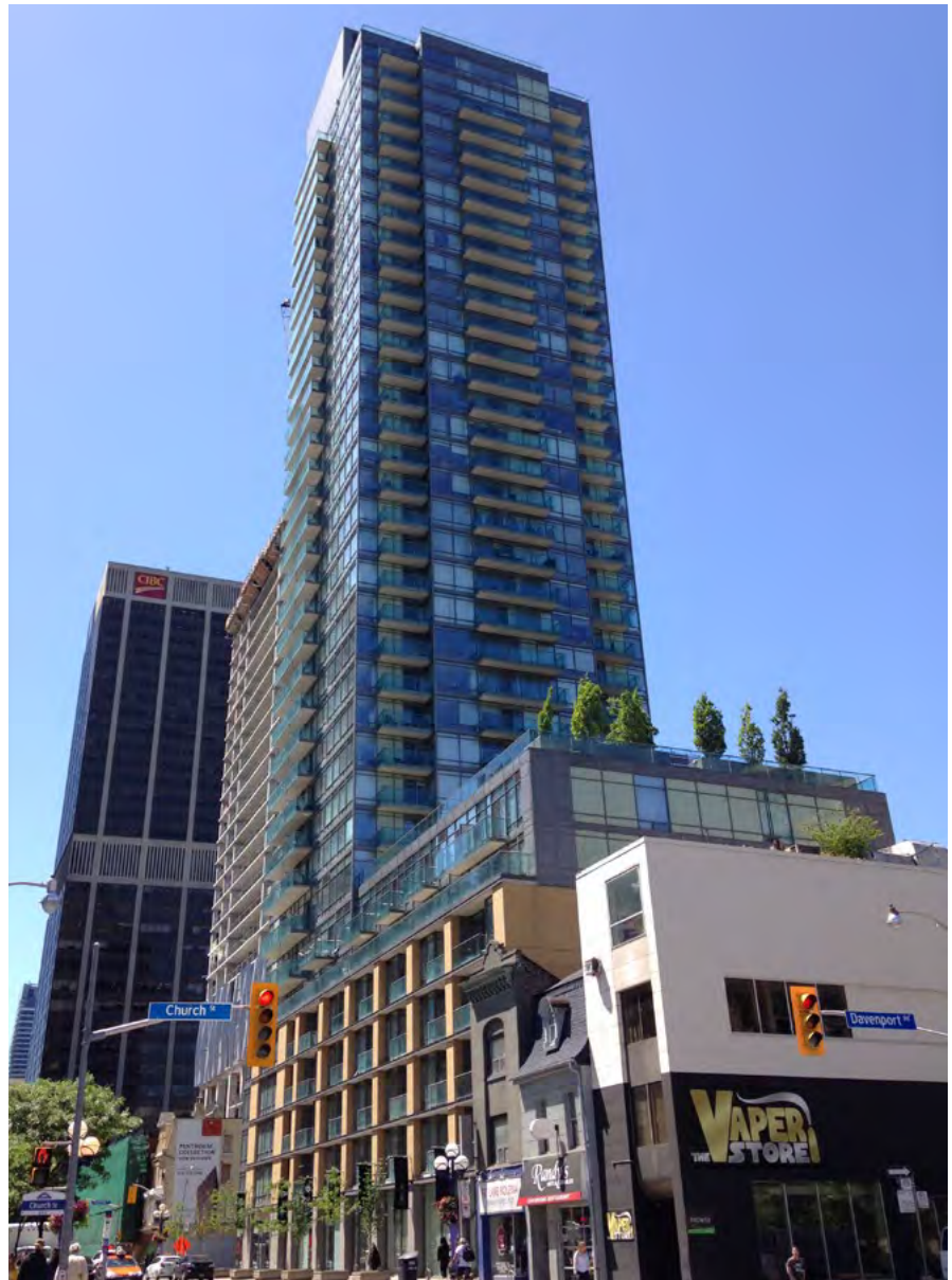
Figure 5.47: Building form transitioning between low- to mid-rise to tall building (Yonge Street and Scollard Street)
