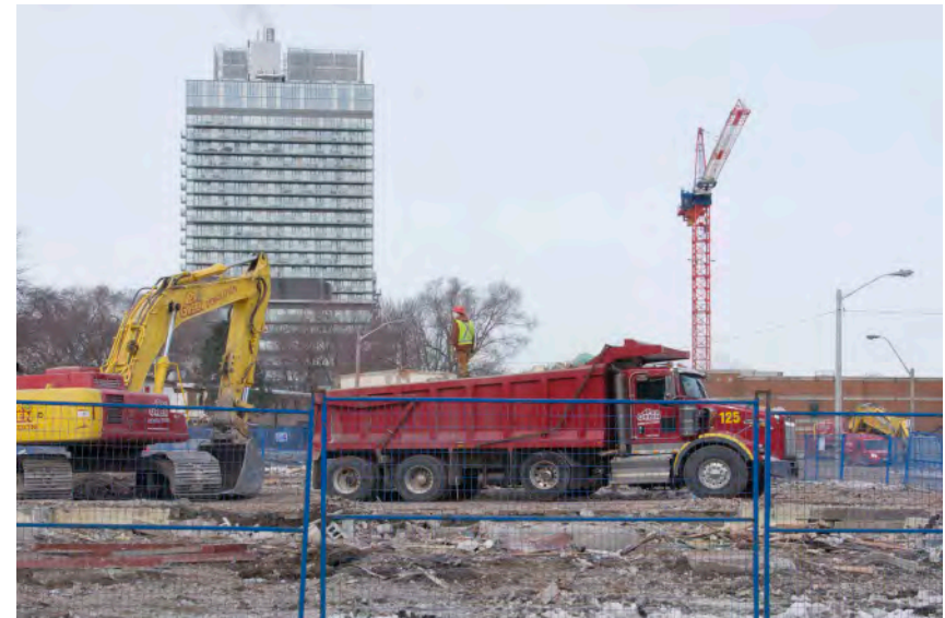
Construction will be phased and coordinated to ensure necessary supporting infrastructure is in place
