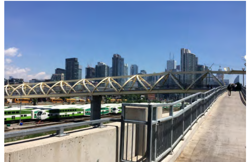
Puente De Luz pedestrian bridge
