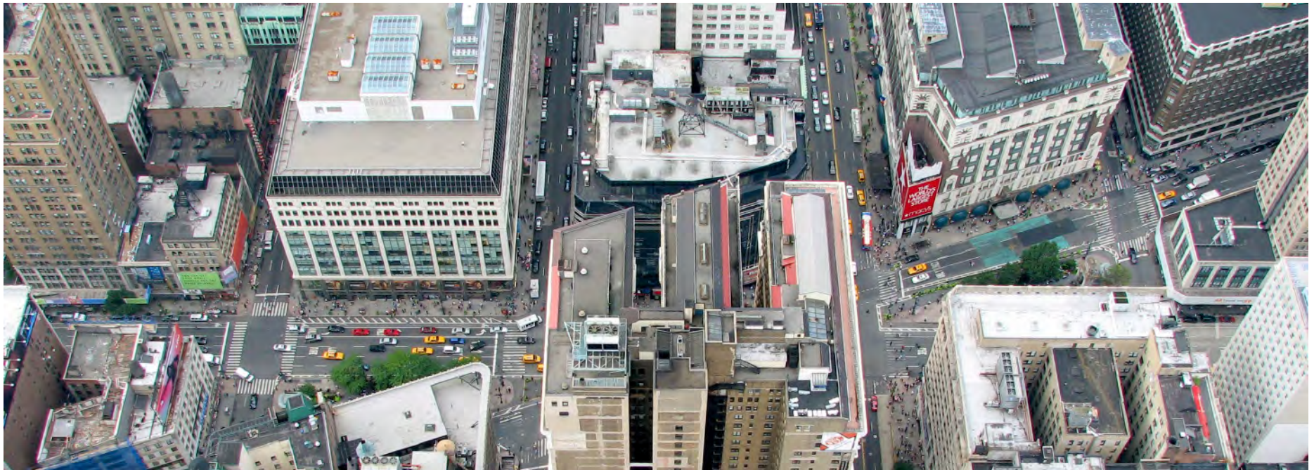
Building faces align to the diagonal orientation of Broadway in New York City
