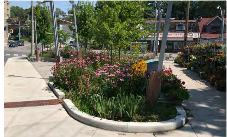
Low Impact Stormwater Management integrated into the streetscape
