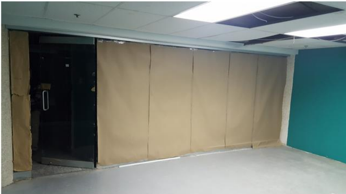
Interior view of Unit 8 at 222 Spadina Avenue
