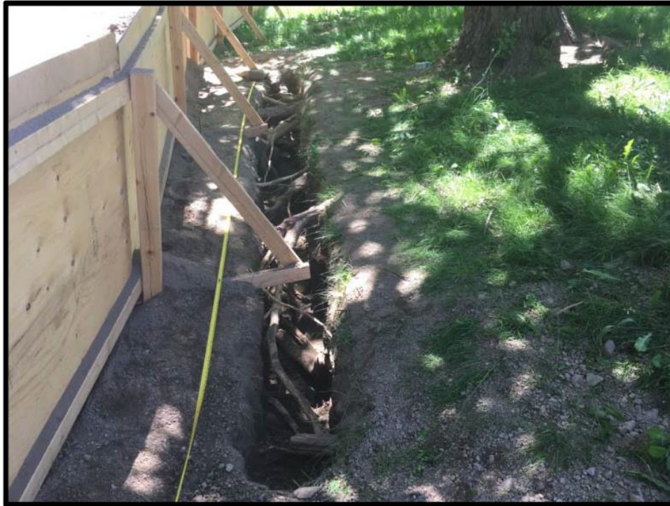
Tree Root Exploration Trench: After surface excavation, a vacuum removes soil to expose tree roots.
