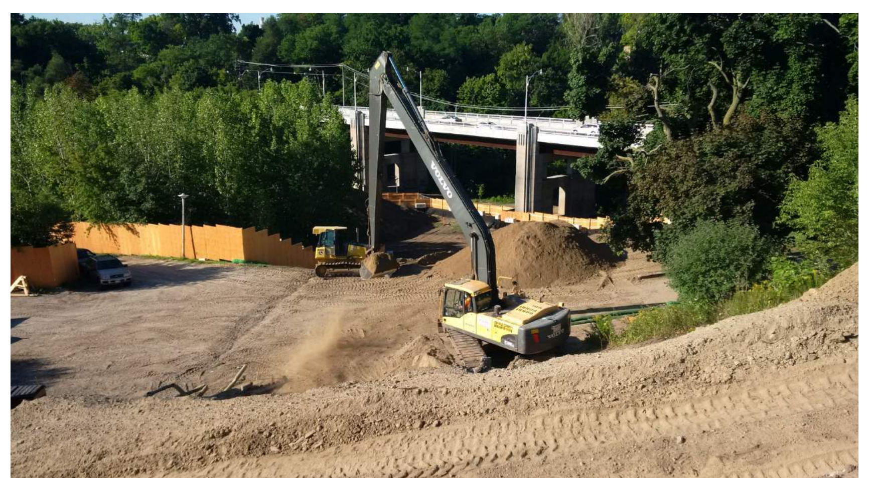
Facing south towards the Spadina Road Bridge, these photos show the proposed DOLA location as a grassed area prior to the rehabilitation project, and as the soil storage area during the project.
