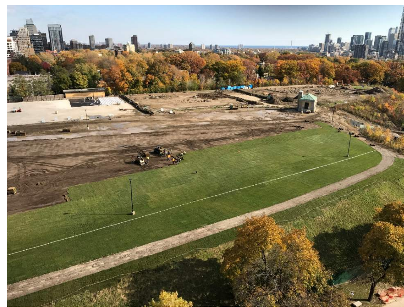
Re-sodding and landscaping of the park area
