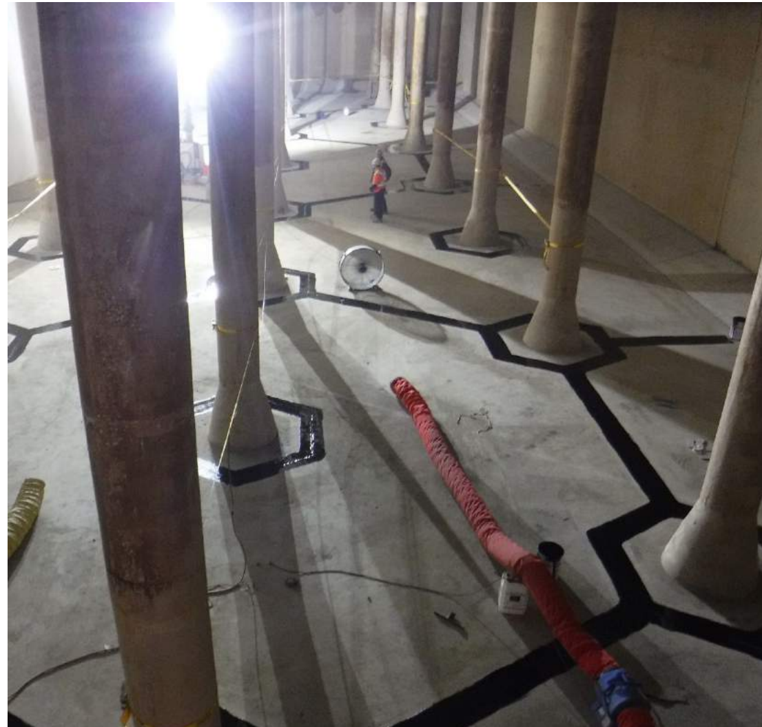
Rehabilitation of the interior of the portal building, valve house and reservoir, including concrete repair and valve replacement
