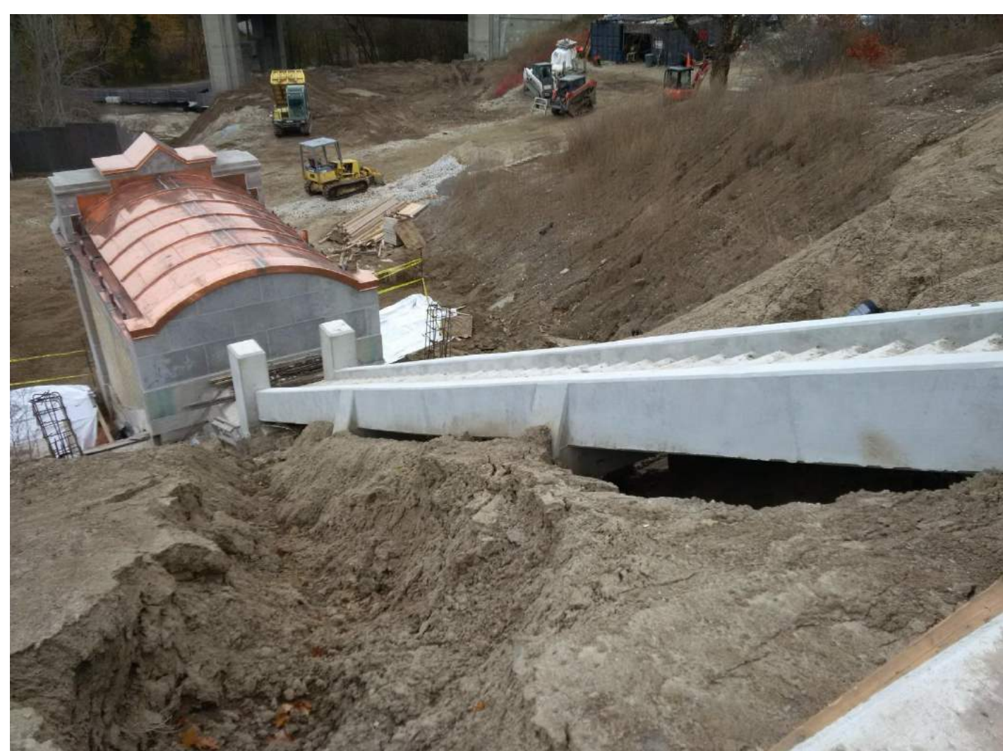
Exterior repairs to the Portal Building and Valve House and replacement of the exterior staircase
