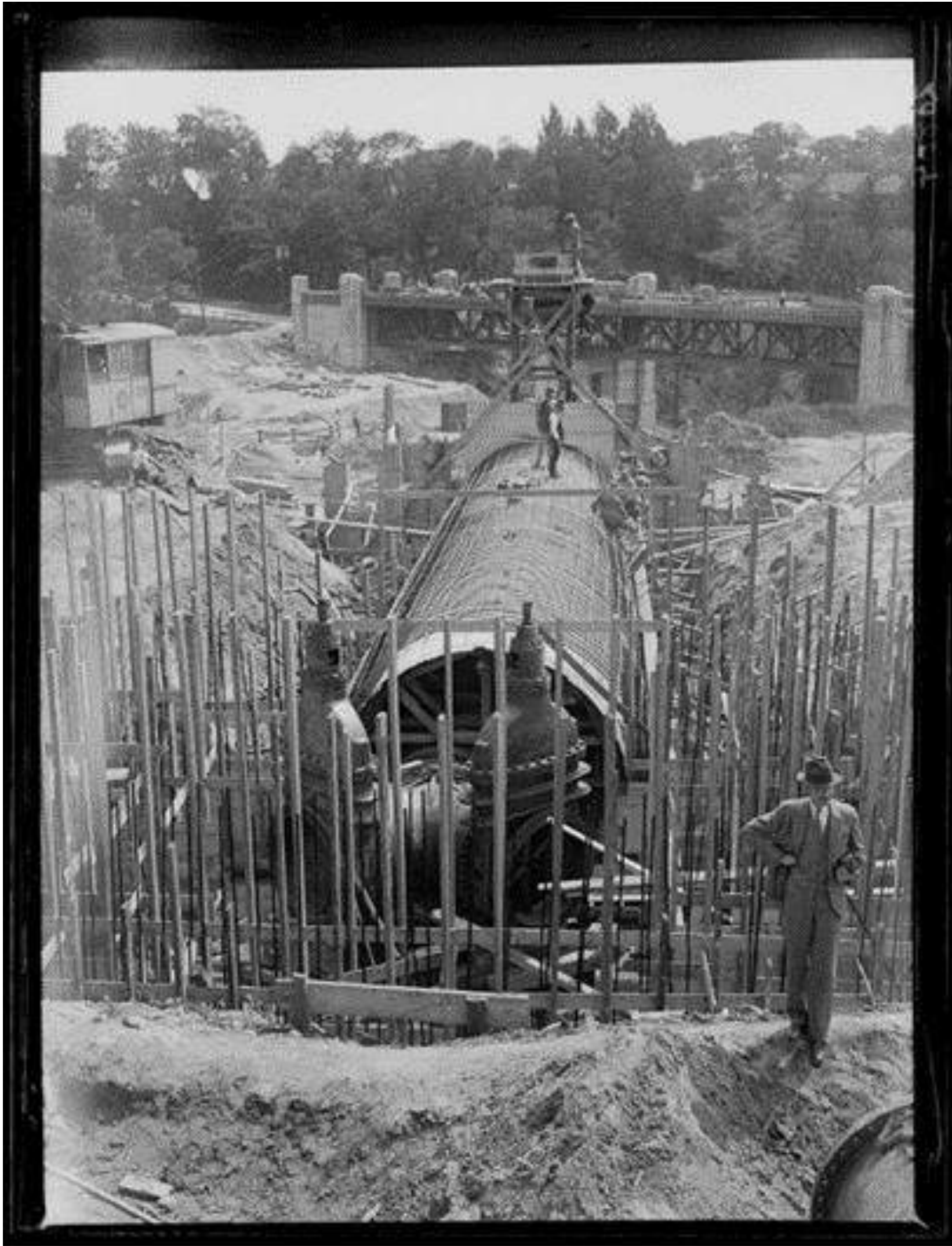
1930: St. Clair Reservoir during construction
