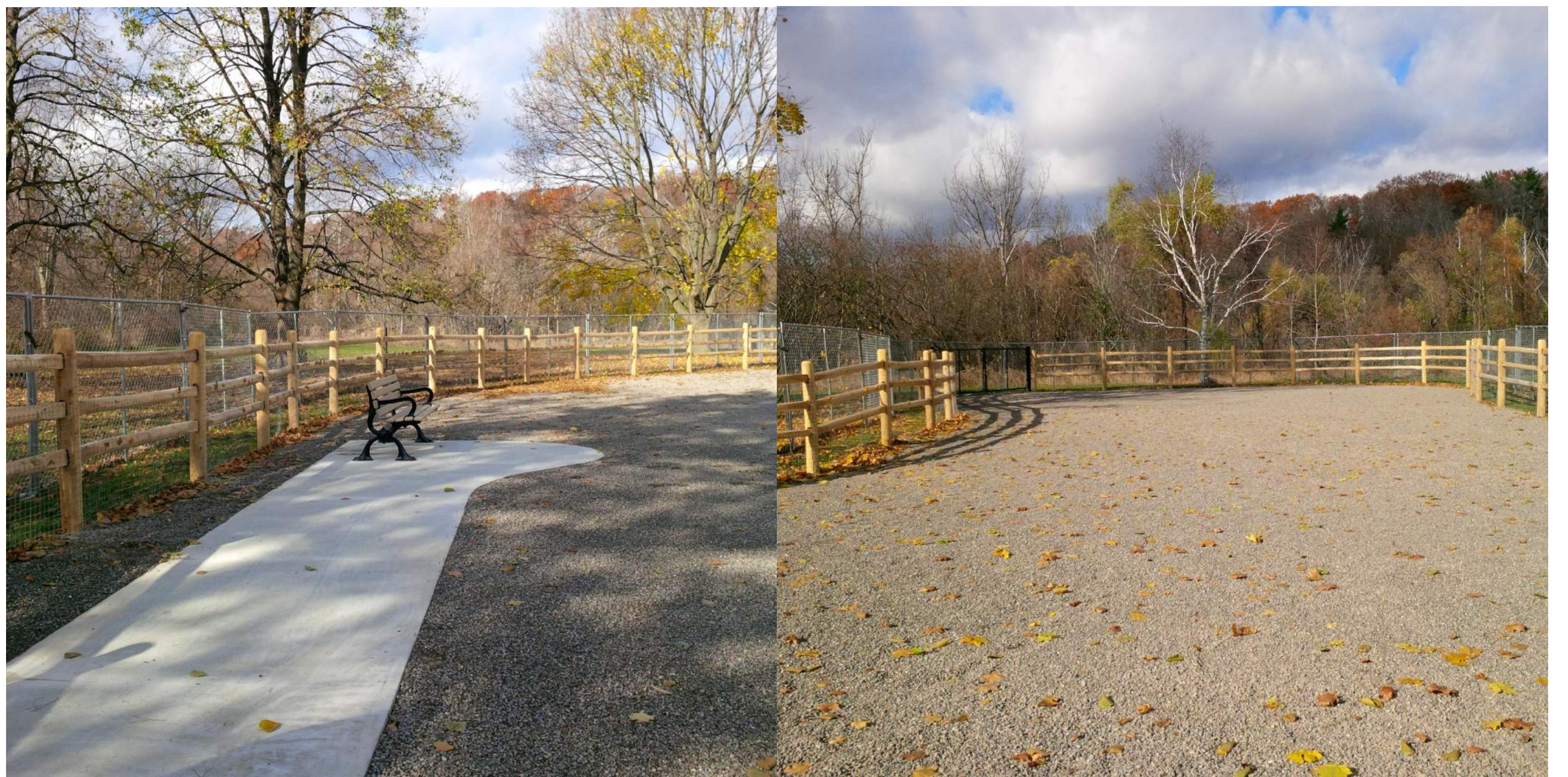
Example of a recently constructed DOLA in a ravine setting in Colonel Danforth Park (*chain link construction fence is temporary and is removed when DOLA opens)
