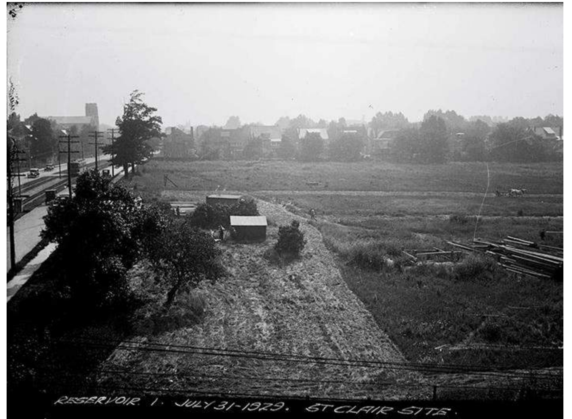
1929: St. Clair Reservoir site prior to construction
