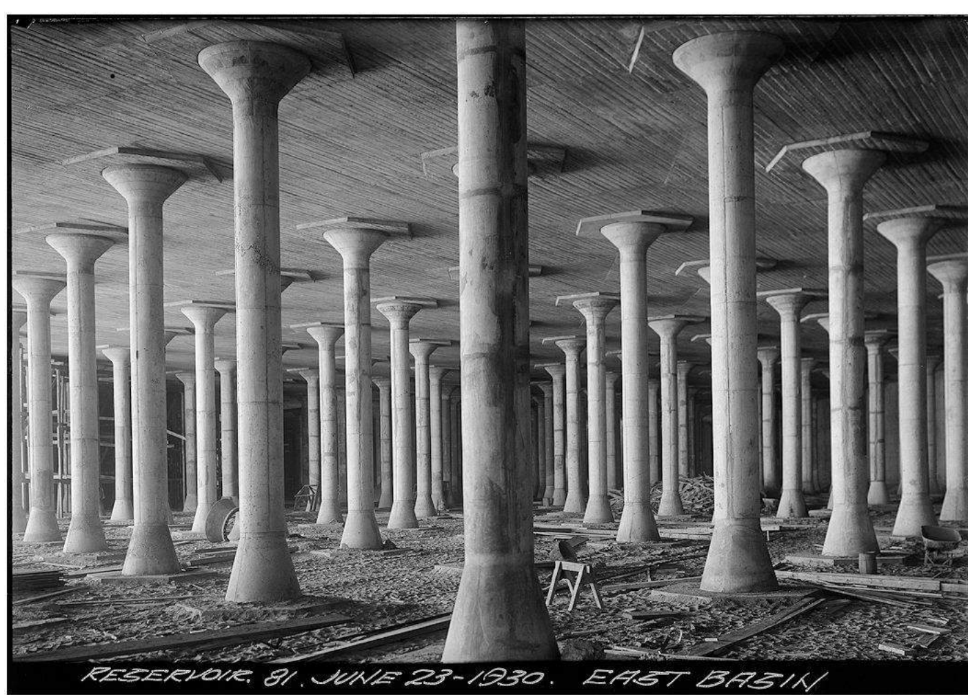
Interior of reservoir under construction
