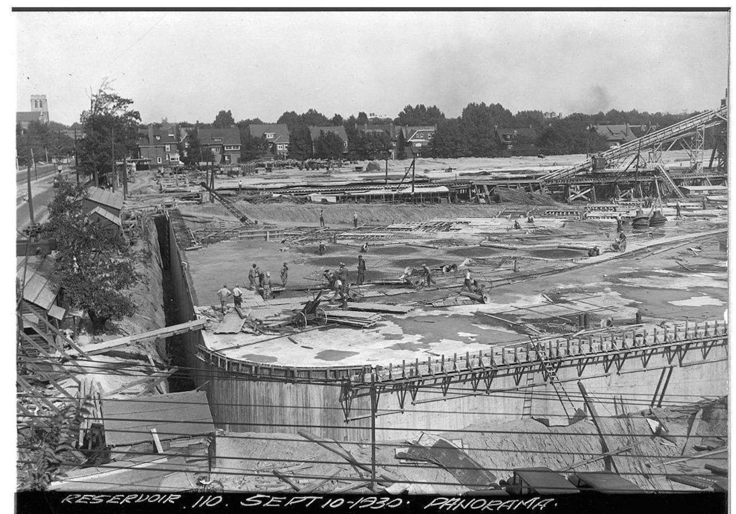
Reservoir under construction in 1930
