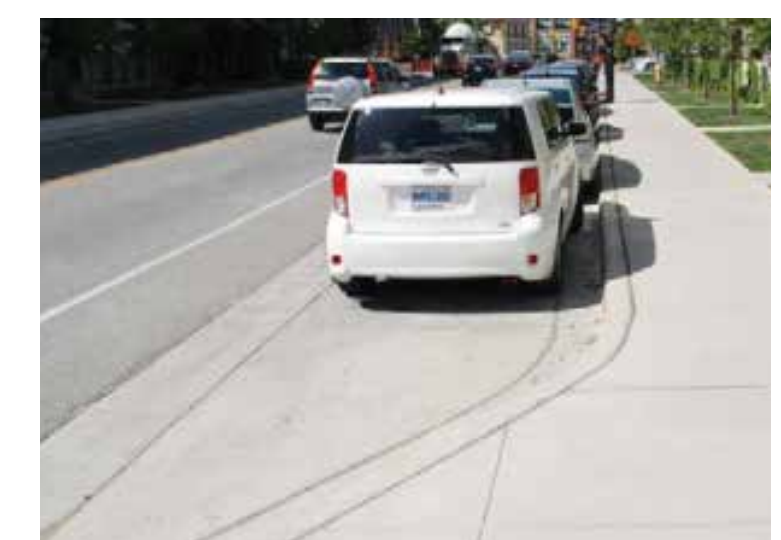
Example of layby parking
