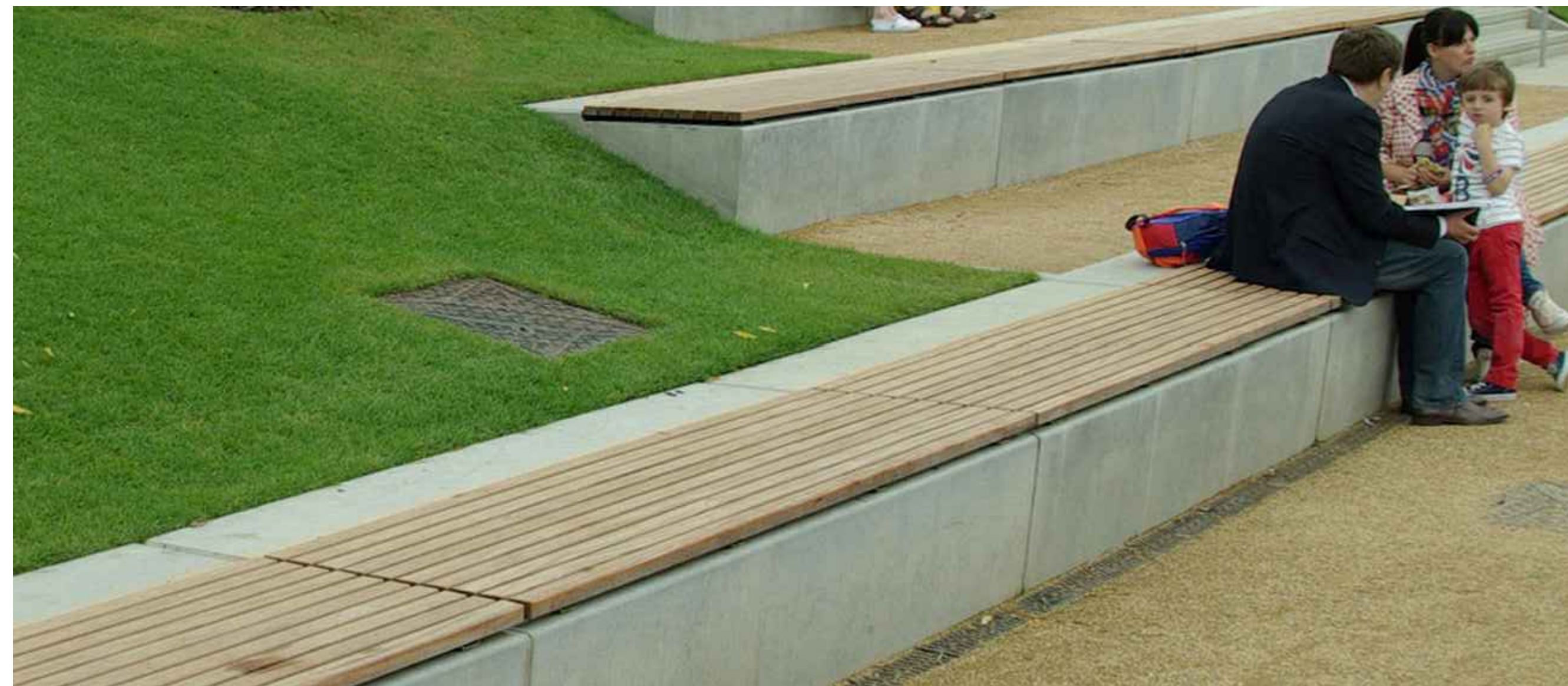
CONCRETE WALL WITH WOOD SLAT TOP
