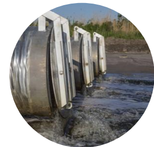
Example of backwater prevention.
