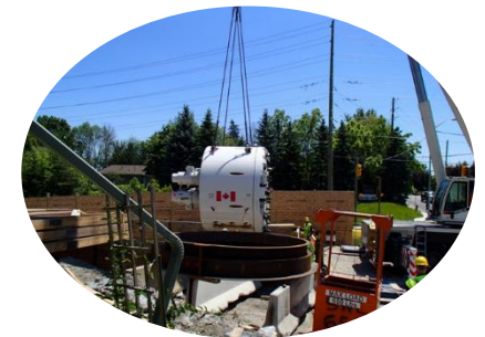
Example of tunnel construction site.
