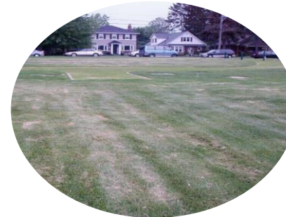
Example of underground storage with surface area landscaped to pre-construction conditions.
