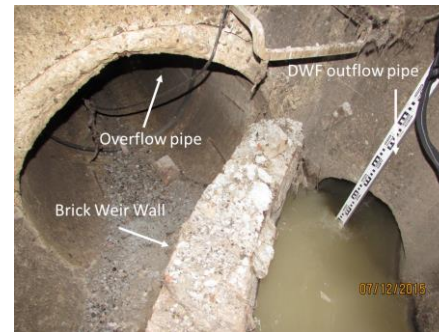
Overflow structure of the Mt. Dennis combined trunk sewer
