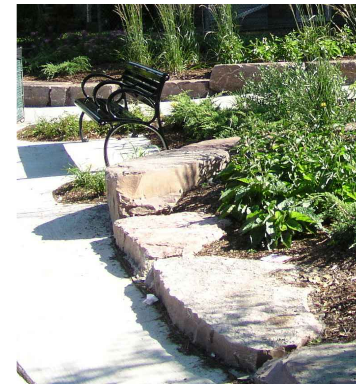
ARMOURSTONE SEAT WALL
