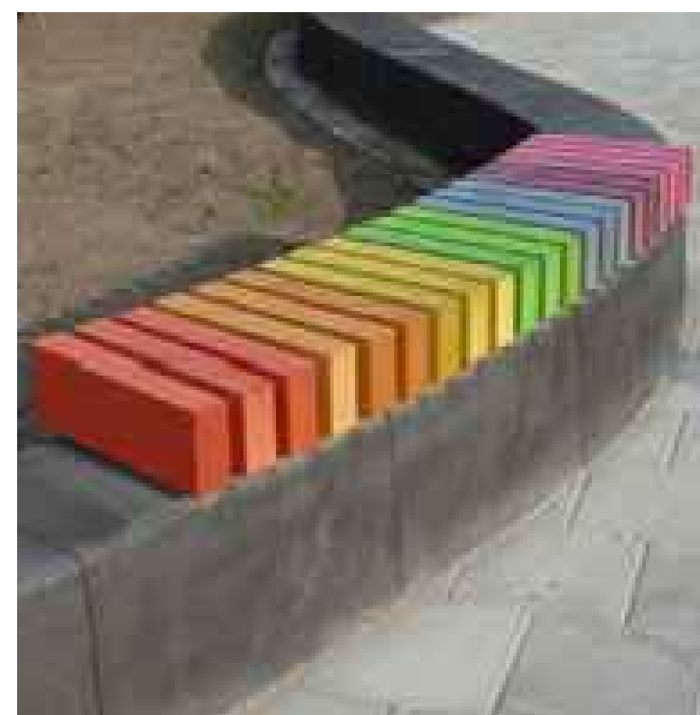
CONCRETE WALL WITH BRIGHTLY COLOURED WOOD SLAT TOP
