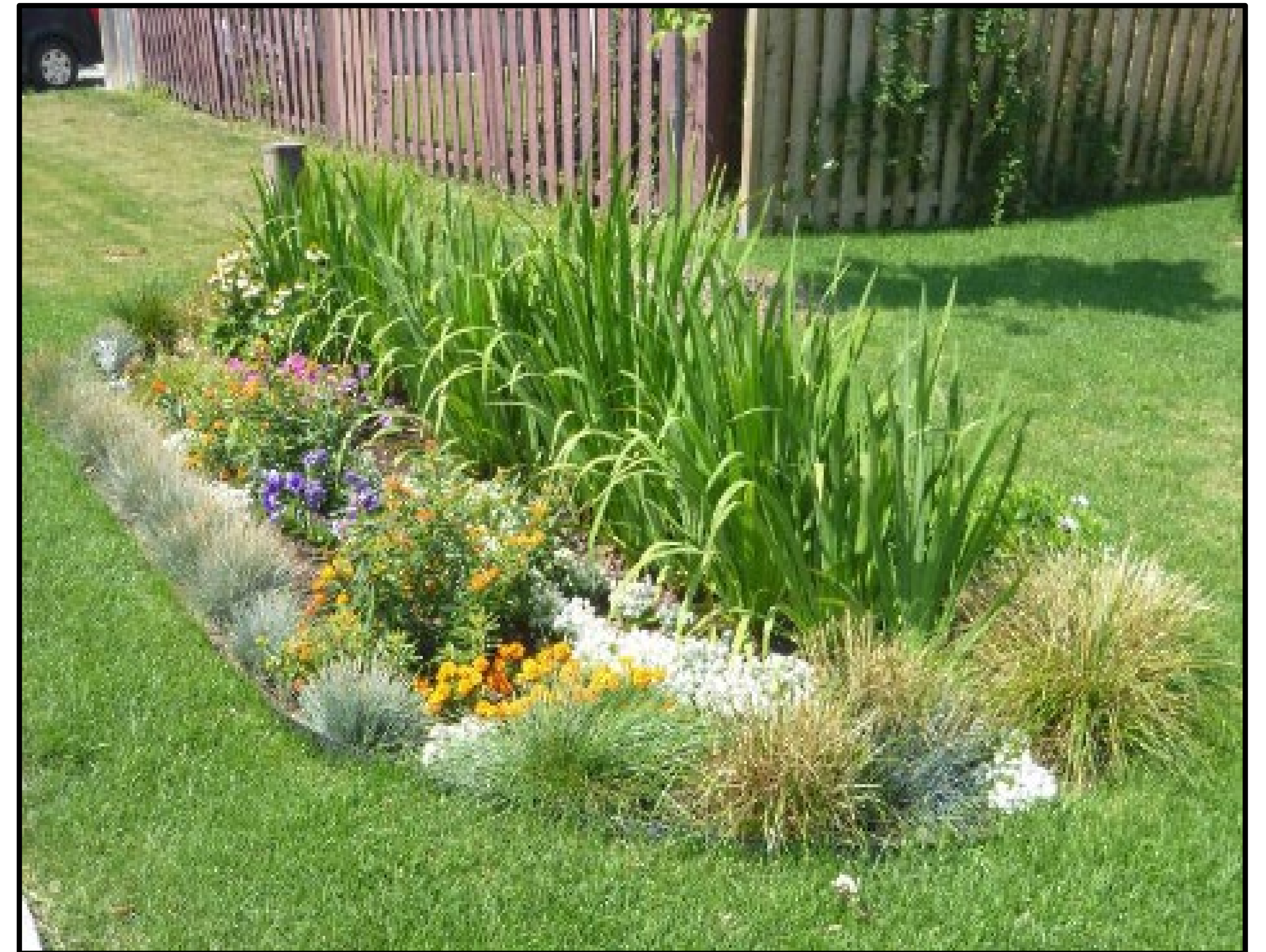
Green Infrastructure Example: Bioretention Cell
