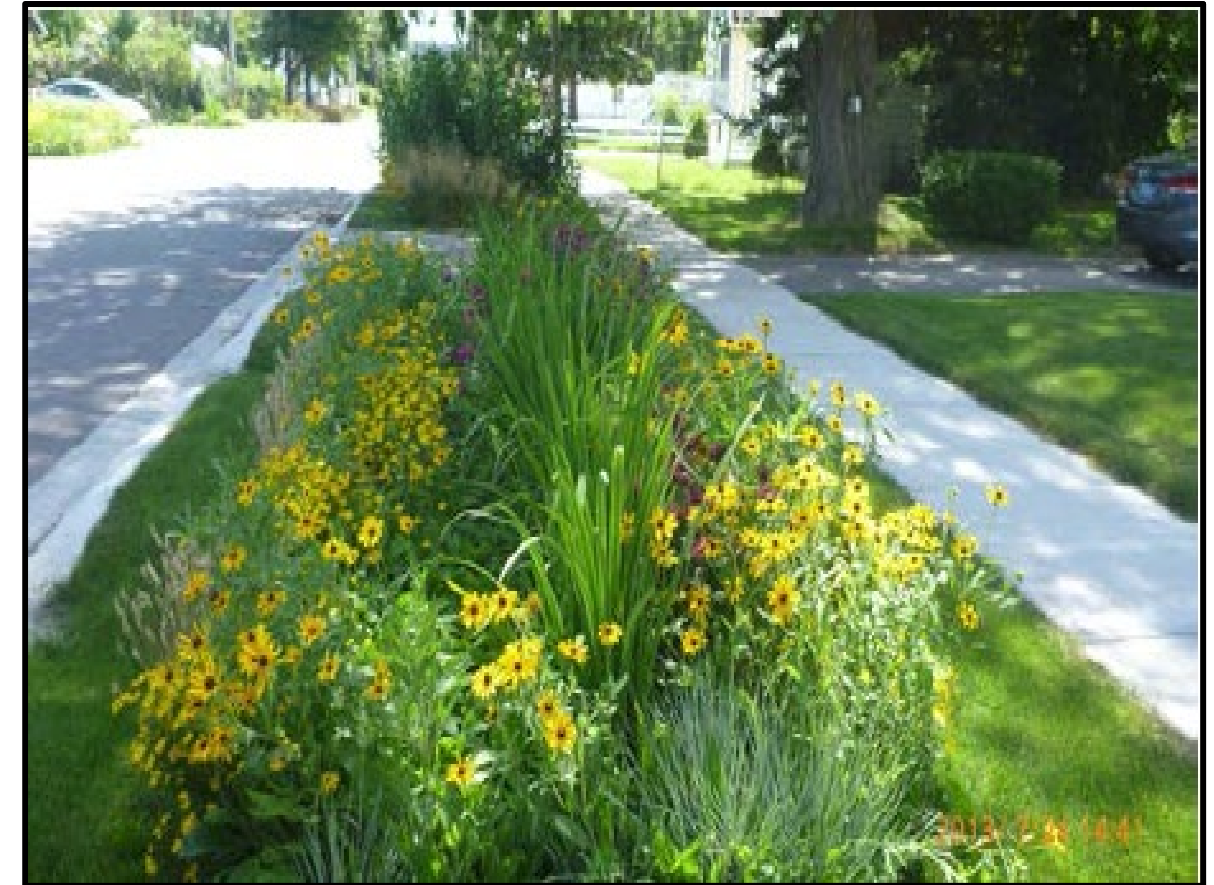
Green Infrastructure Example: Bioswales for ditched roads
