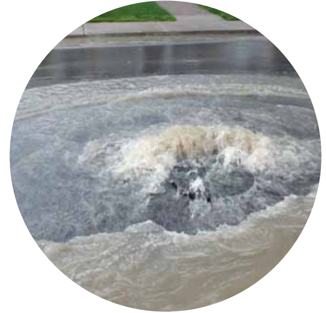
Example of sanitary trunk sewer overflow during a wet weather event
