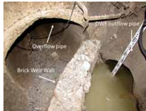
Overflow structure of the Mt. Dennis combined trunk sewer
