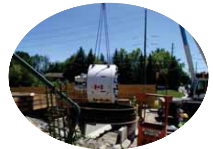
Example of tunnel construction site.
