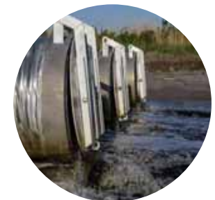
Example of backwater prevention.
