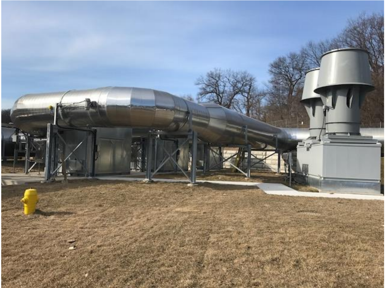
Figure 1: The Central Biofilter fans
