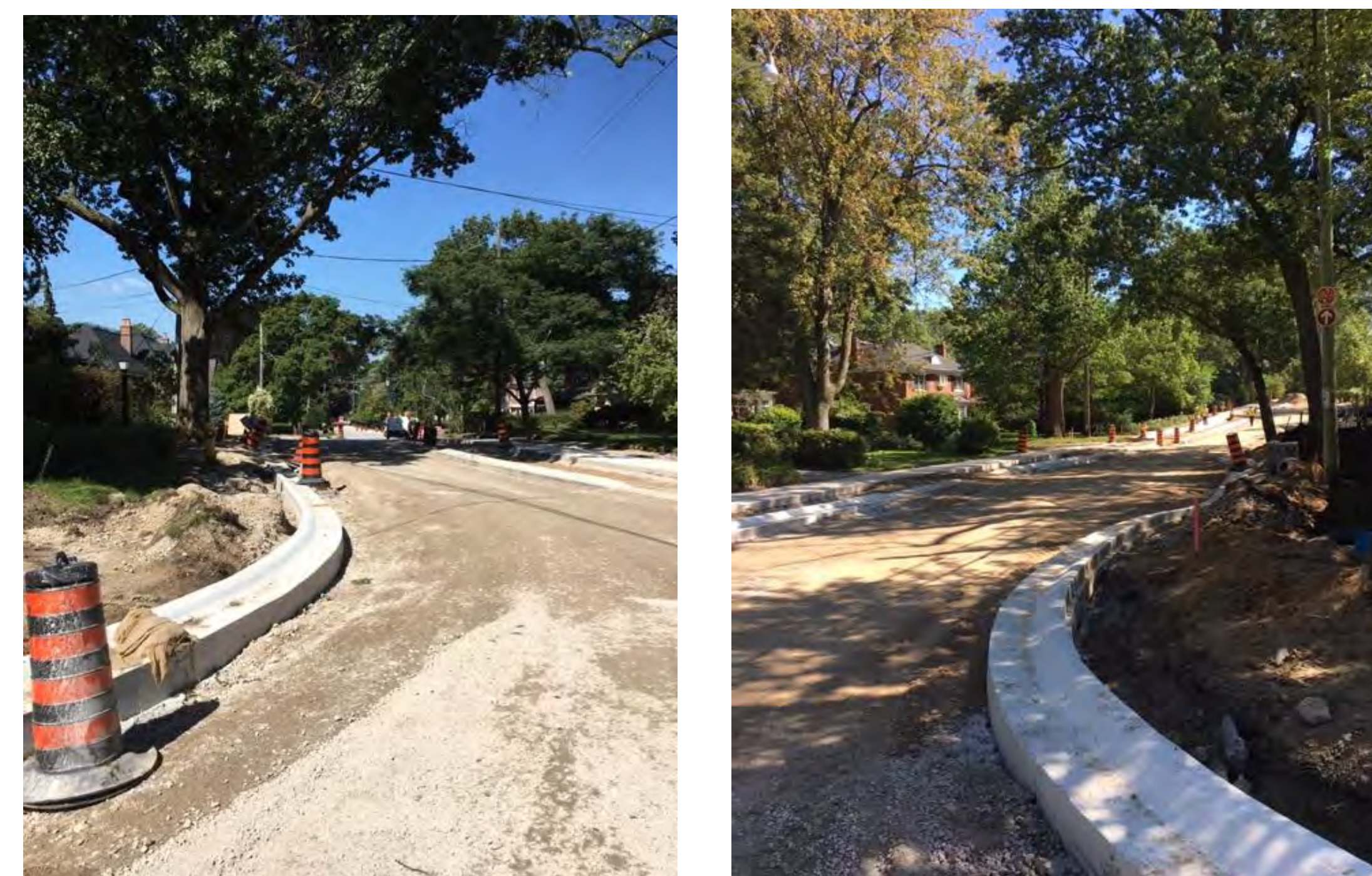
Example of road reconstruction
