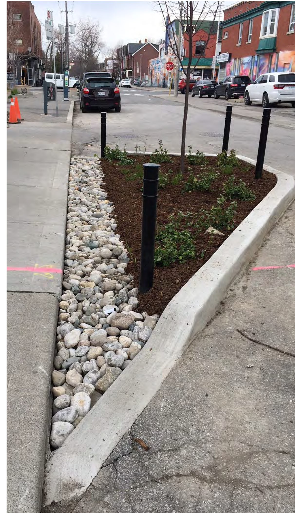
Curb extension at Concord Avenue & Bloor Street
