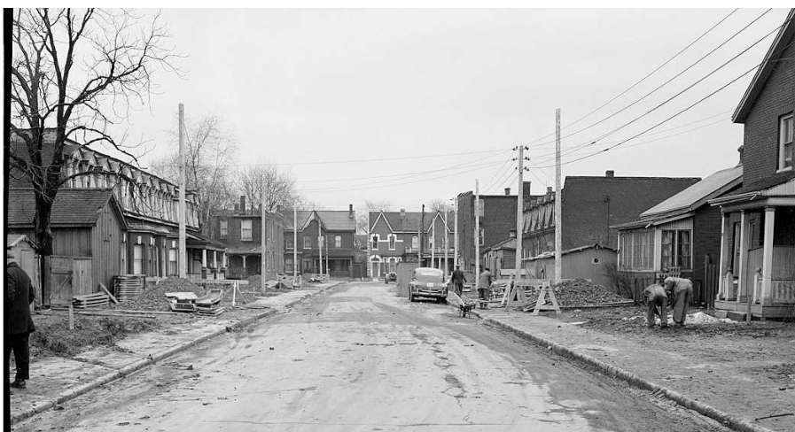
Construction of Peel Ave. & Gladstone Ave., 1949
