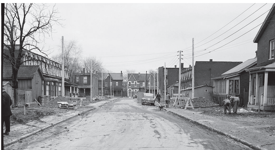
Construction of Peel Ave. & Gladstone Ave., 1949
