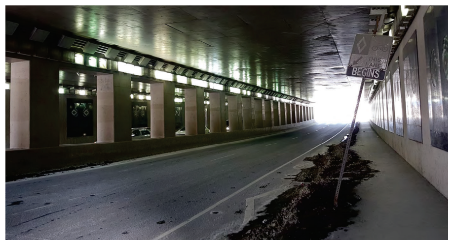
Look through the Dufferin underpass. 2019
