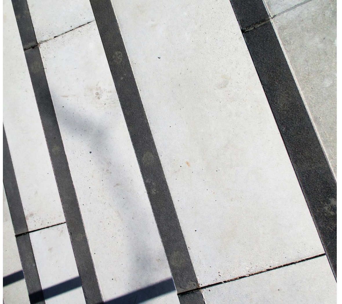
Precast concrete steps with black nosing strip flush to front edge
