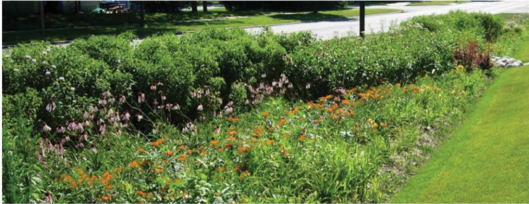
Range of plantings possible within bioswale structure, below which a pipe drains away excess water
