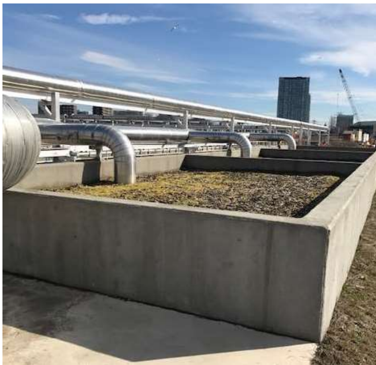
Figure 3: The South Biofilter
