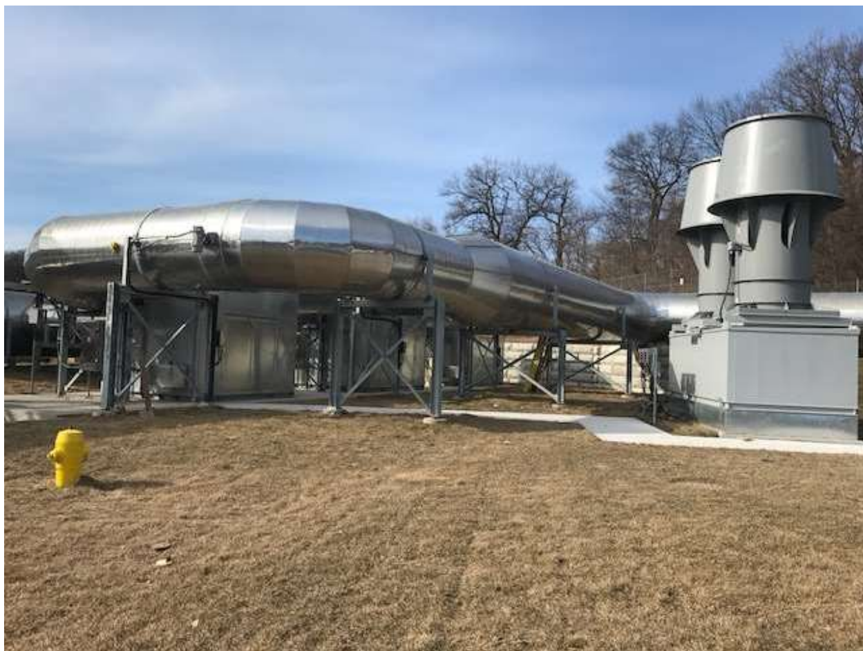
Figure 1: The Central Biofilter fans
