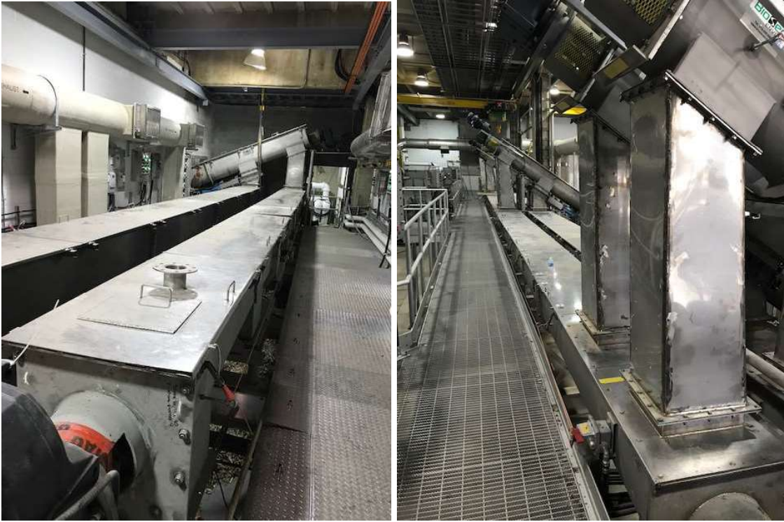
Figure 4 The new headhouse loading bay (left) and screenings conveyor systems (right)
