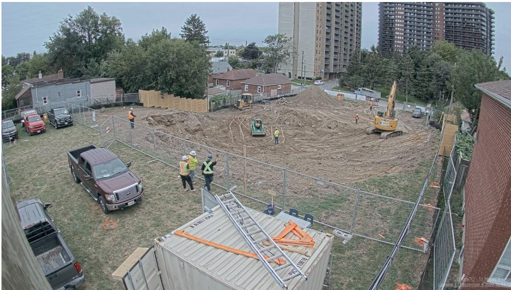
Figure 1- Site Preparation Underway at 11 Macey Avenue
