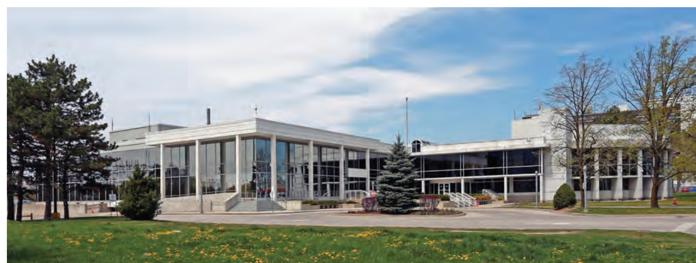
Former Hydro-Electric Commission Building, built in 1963
