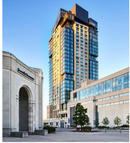
The district energy system at Exhibition Place provides heating and cooling to the new Hotel X Toronto.
