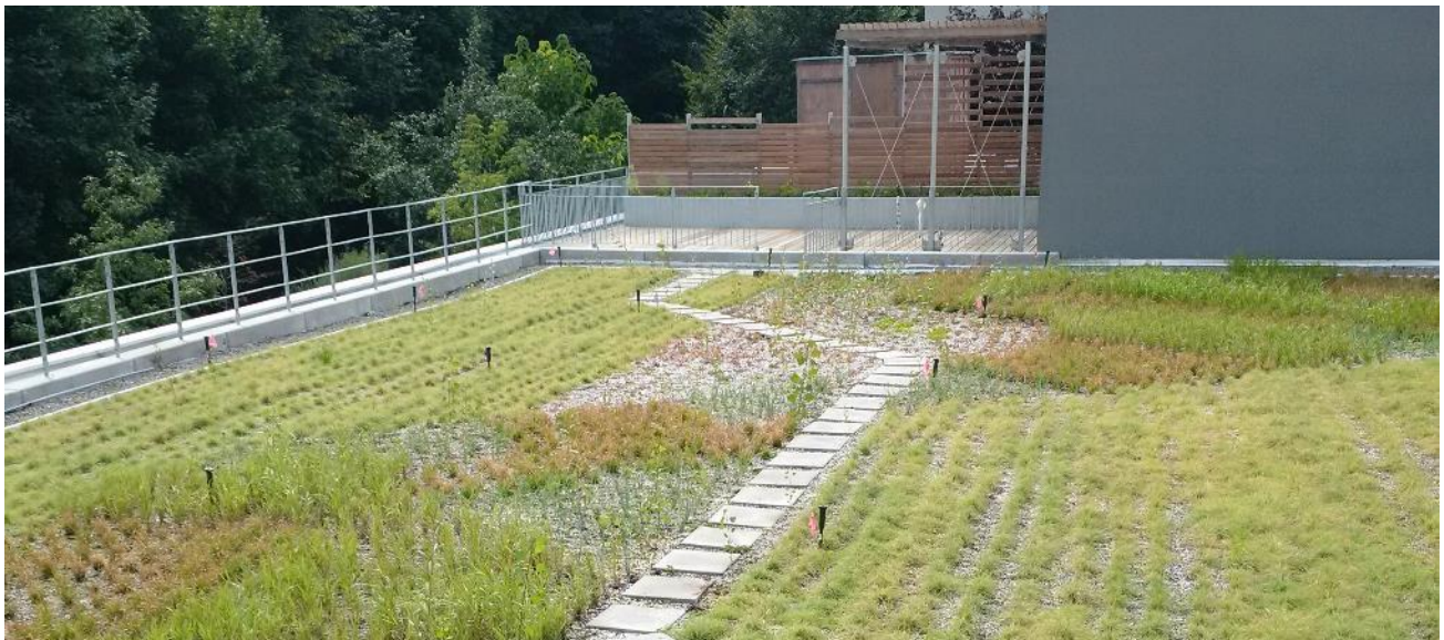
Green Roof installed by Eco-roof Incentive Program participant
