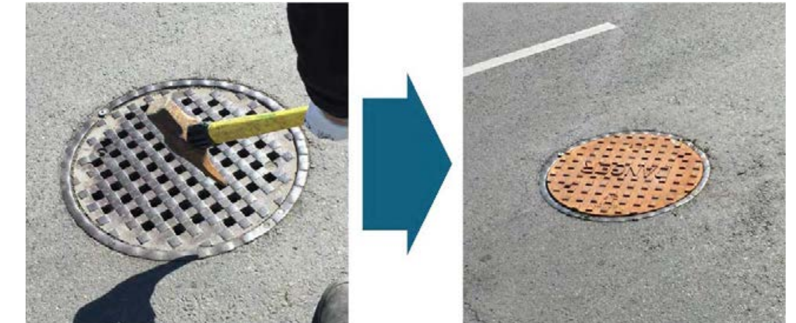
Example of maintenance hole cover replacement.
