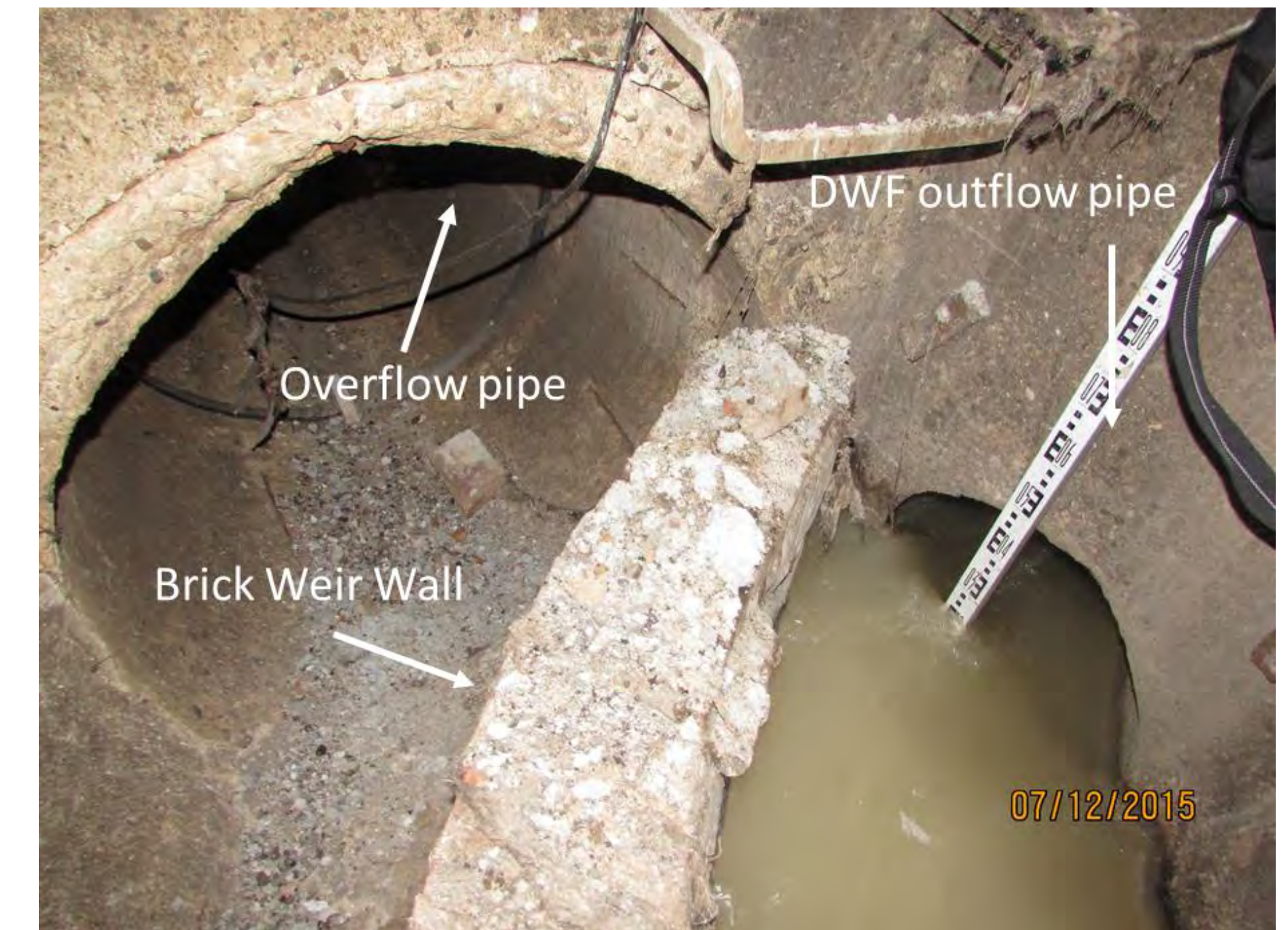
Overflow structure of the Mt. Dennis combined trunk sewer
