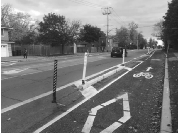
Option A: Concrete curbs and bollards
