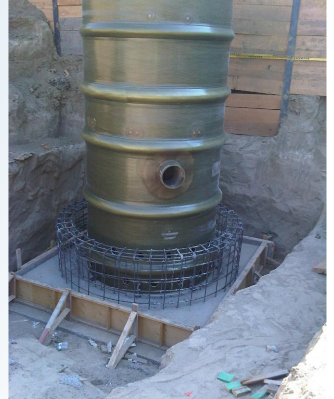
Example of Pre-Packaged Pumping Station Image Source: Barski Industries Ltd.
