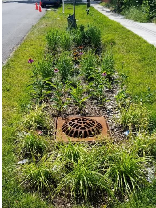
Bioswale example from Byng Ave in Toronto
