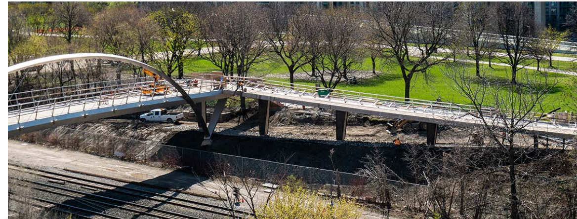
Garrison Crossing Pedestrian & Cyclist Bridge, Toronto, ON
