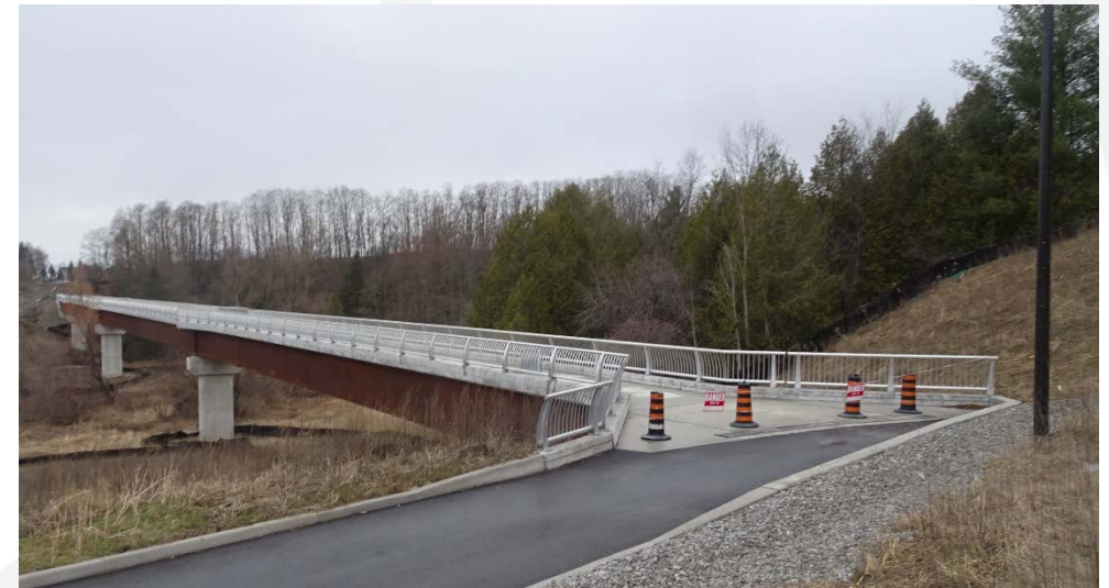
Pine Valley Pedestrian Bridge, Vaughan, ON
