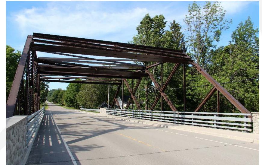
New Creemore Bridge, Clearview Township, ON
