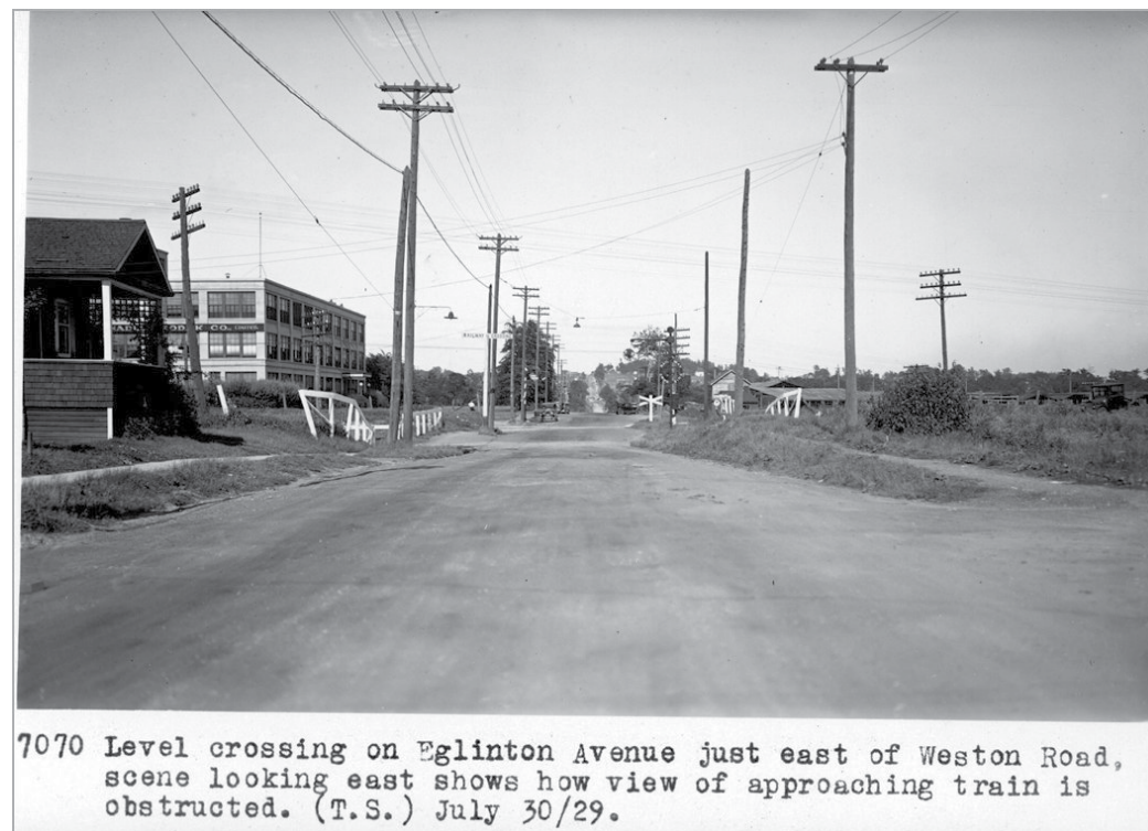
Level crossing, on Eglinton Avenue, just east of Weston Road, scene looking east, shows how view of approaching train is obstructed, (Traffic Study Department)
