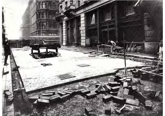
77. Laying of asphalt blocks, a by-product of the gasworks, on Victoria Street (Consumers' Gas, ca.1904)
