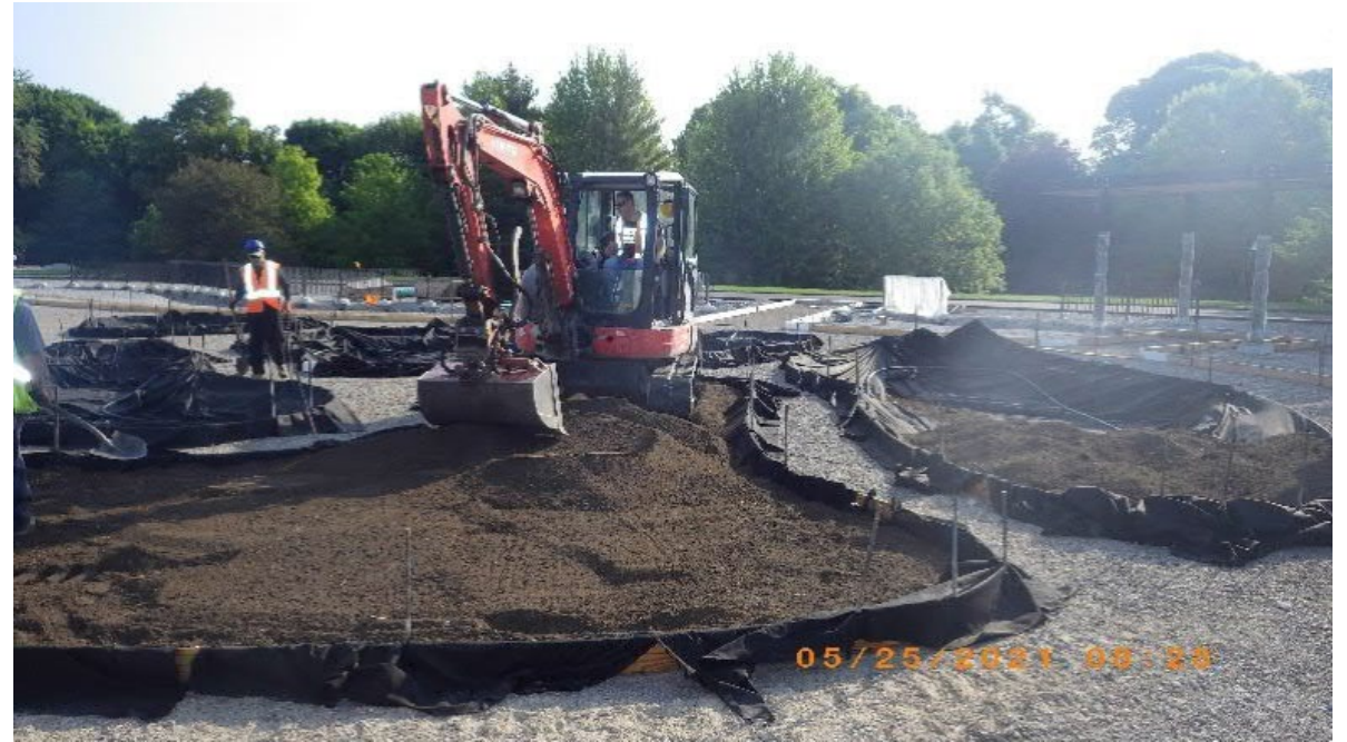
Growing medium installed in the Garden Beds
