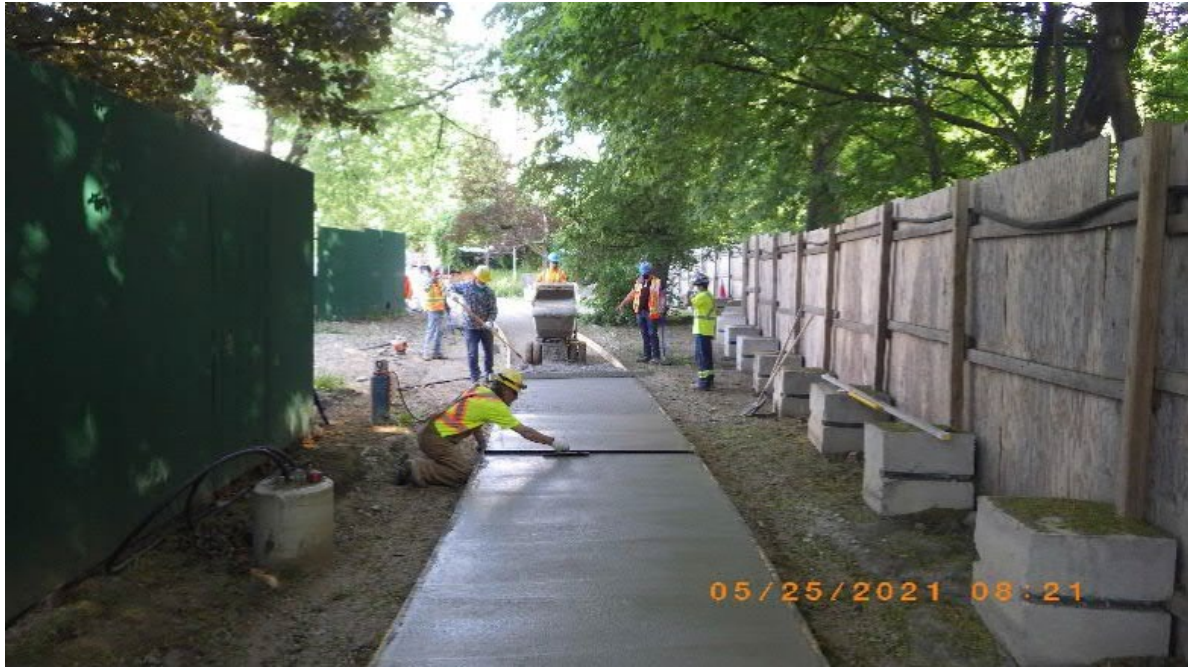
Installing walkways
