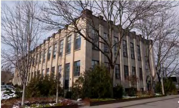
The factory building at 284 St. Helens Avenue is used as residential lofts today (CBCollective 2020).
