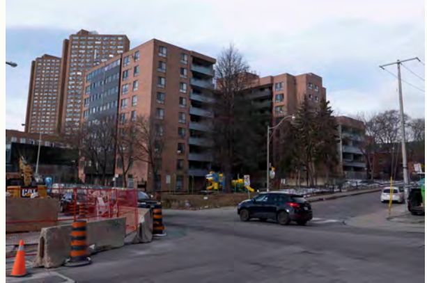
Infill mid-rise residential building at 120 Perth Avenue (CBCollective 2020).
