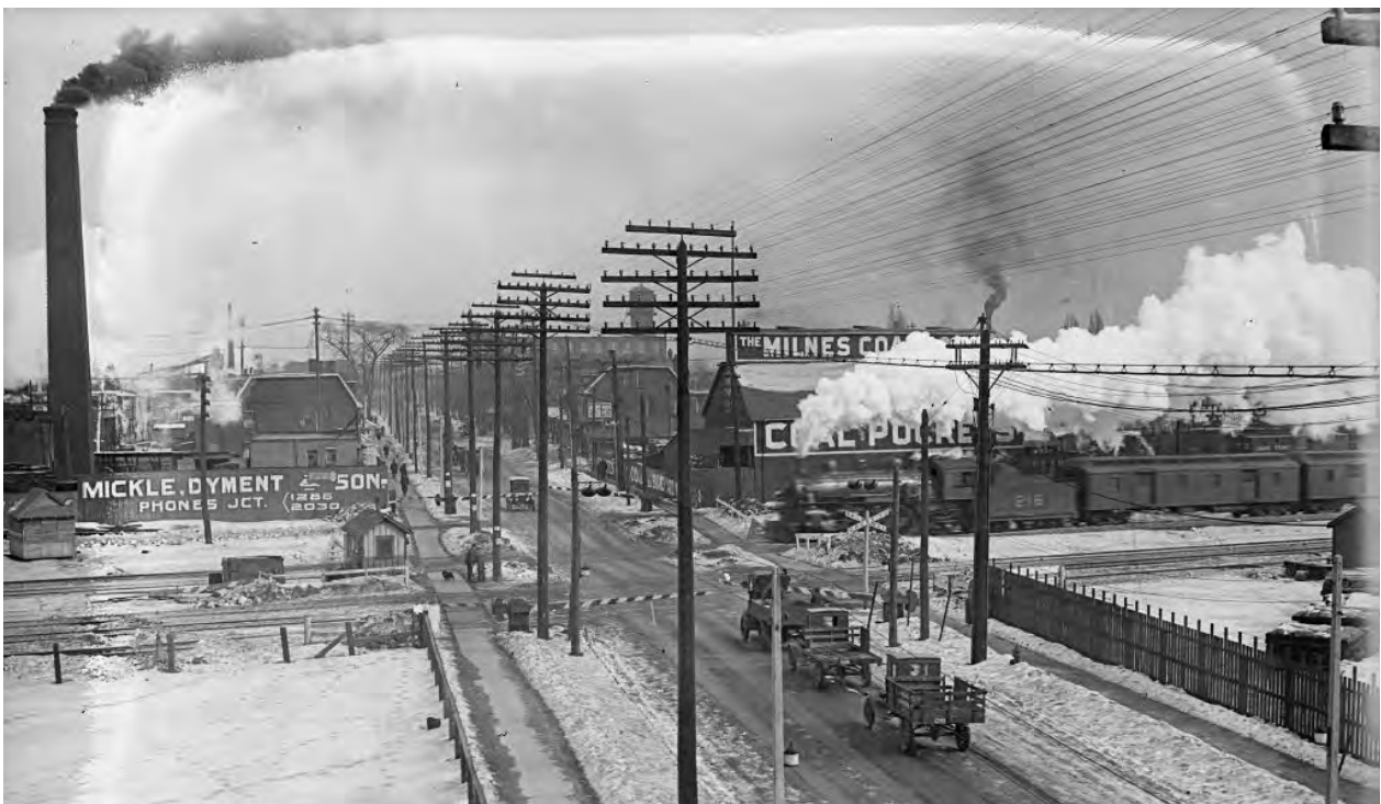
Figure 20: 1923 photograph showing industries east of the CPR corridor, including coal yards at centre-right. The railways' level crossings constituted a constant impediment to traffic through the area along Bloor Street ( City of Toronto Archives: f1266_it0216 ).
