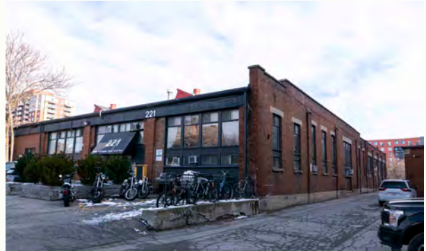
A collection of factory structures at 221 Sterling Road (CBCollective 2020).
