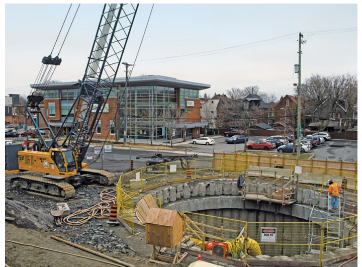
Example of a vertical shaft
