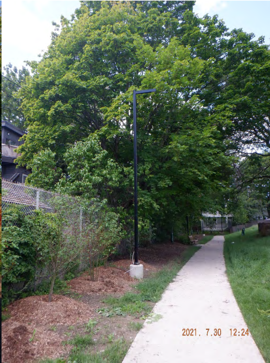
New lighting standards installed west of Valve House (left photo) and south side of park (right photo)
