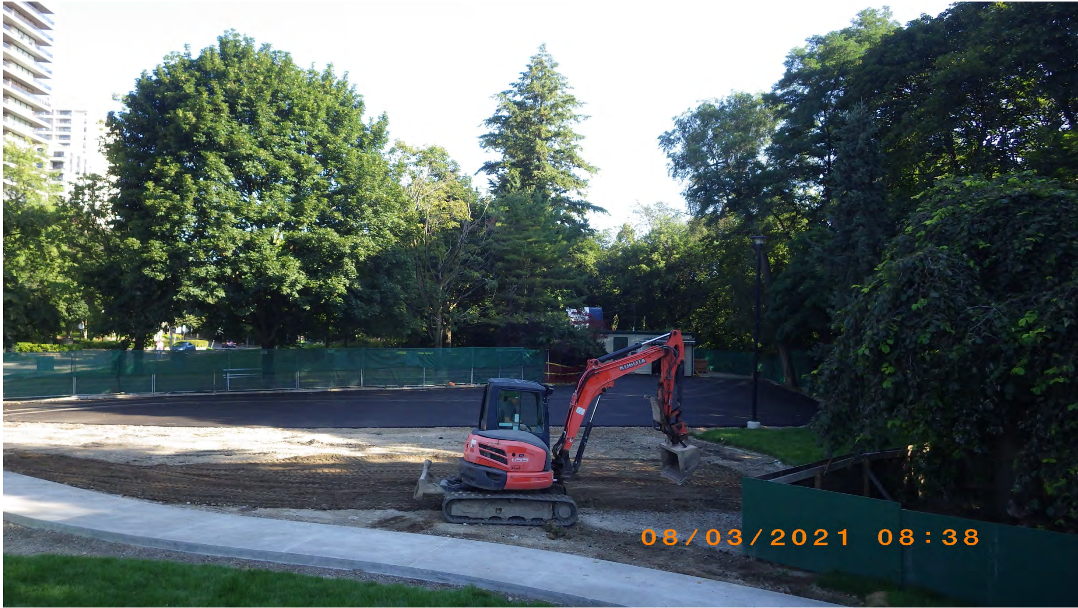
New driveway to the Parks Avoca Yard Building
