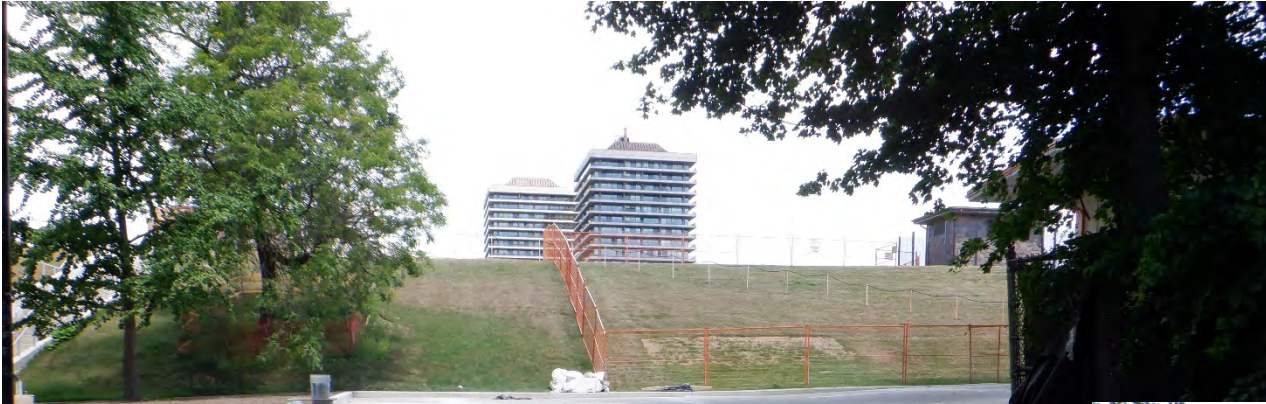
Little park driveway - forms
