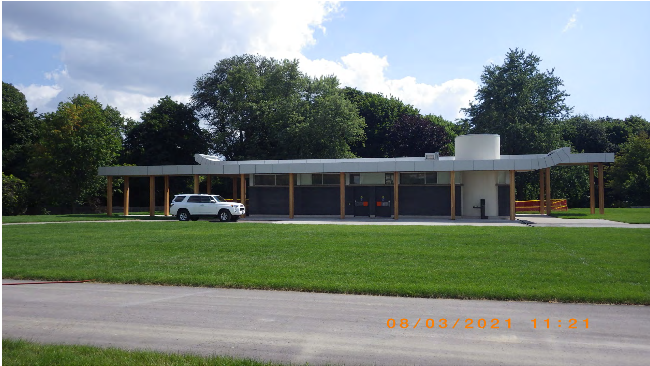
Washroom – west view
