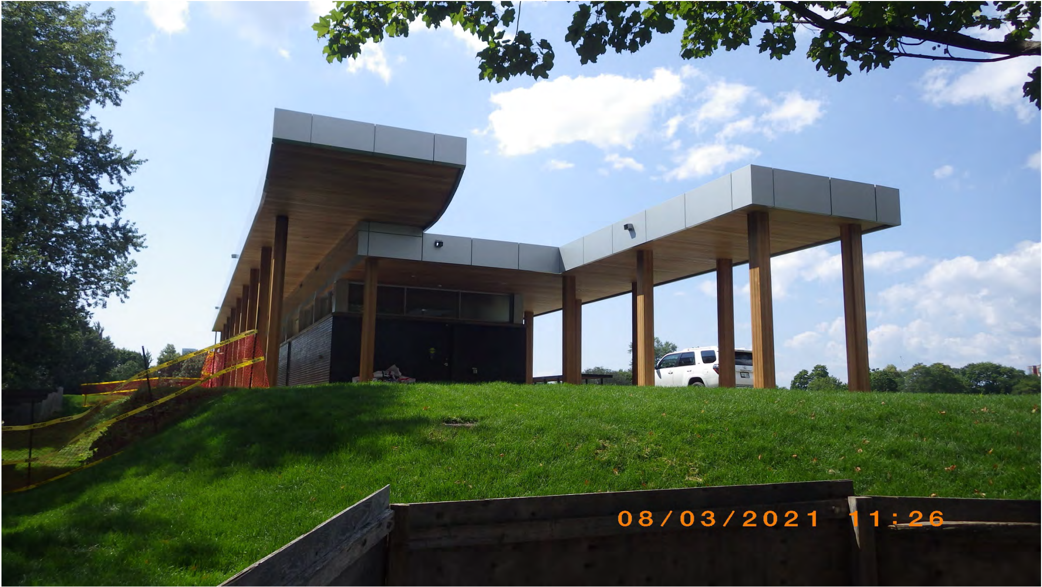
Washroom – north view
