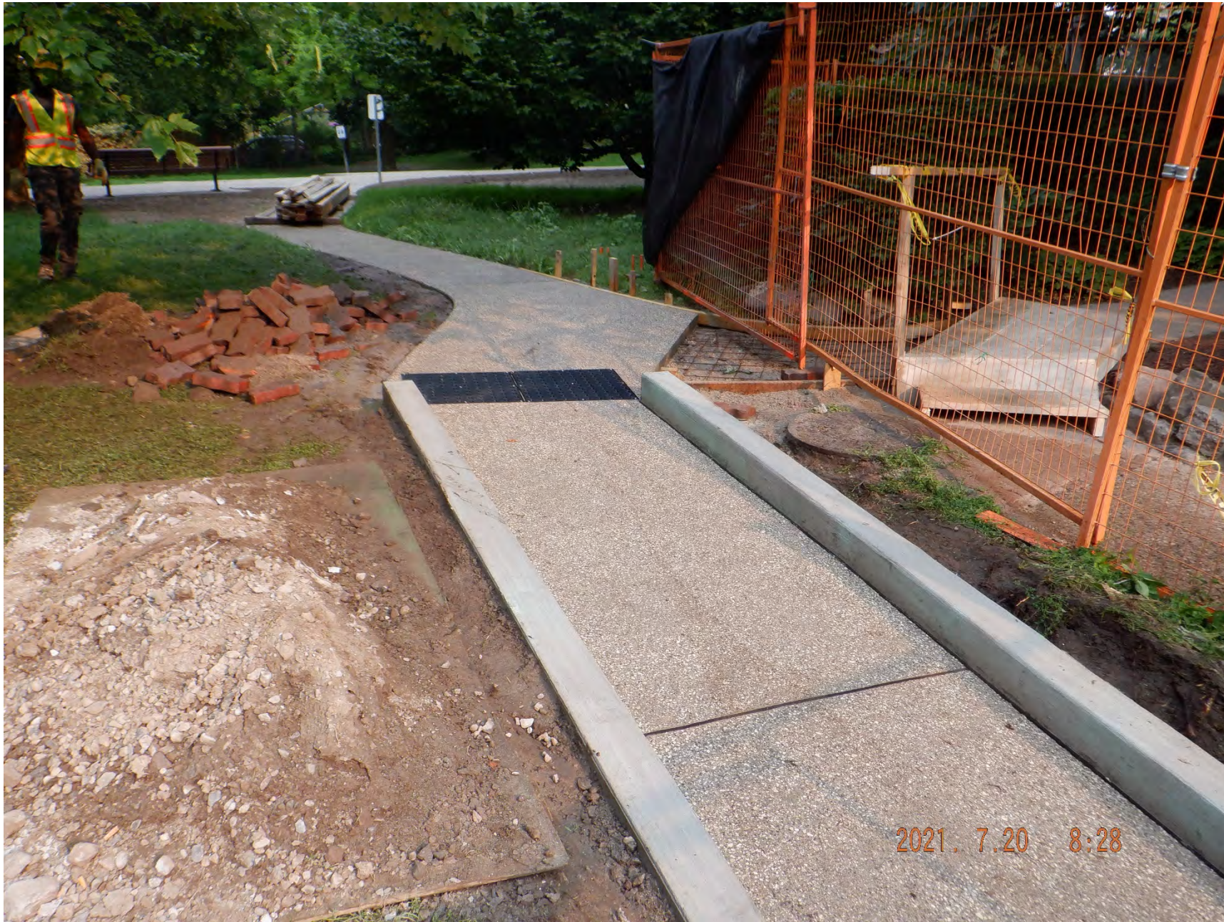
Ramp from Summerhill Gardens, looking west
