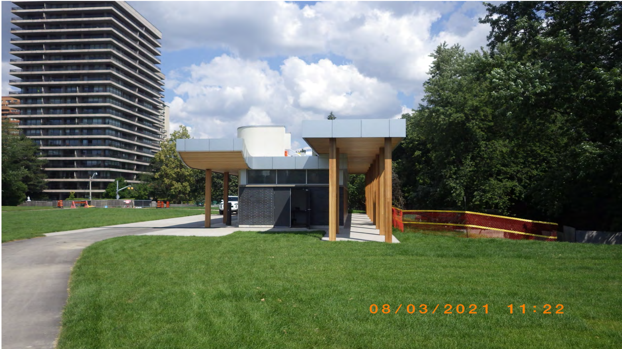
Washroom – south view
