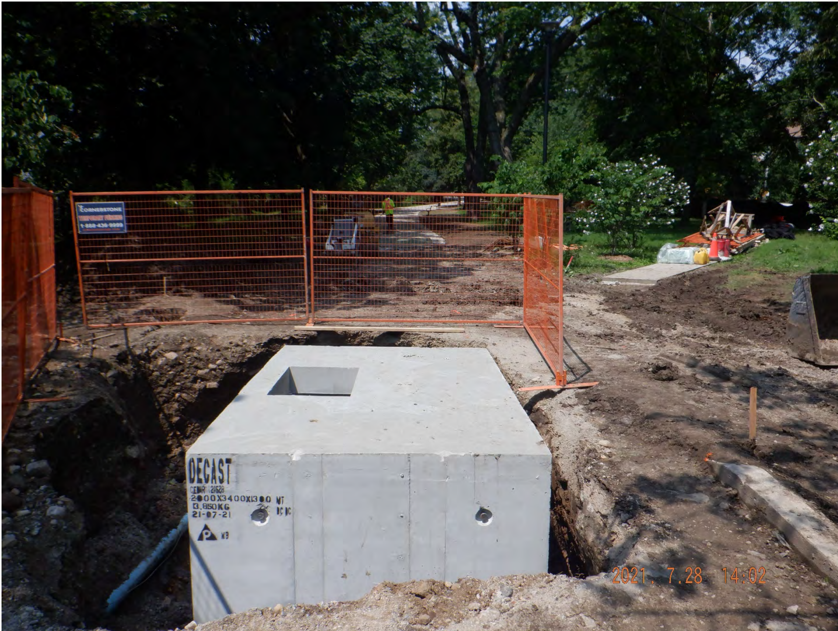
Watermain chamber to service the drinking fountain in Little Park
