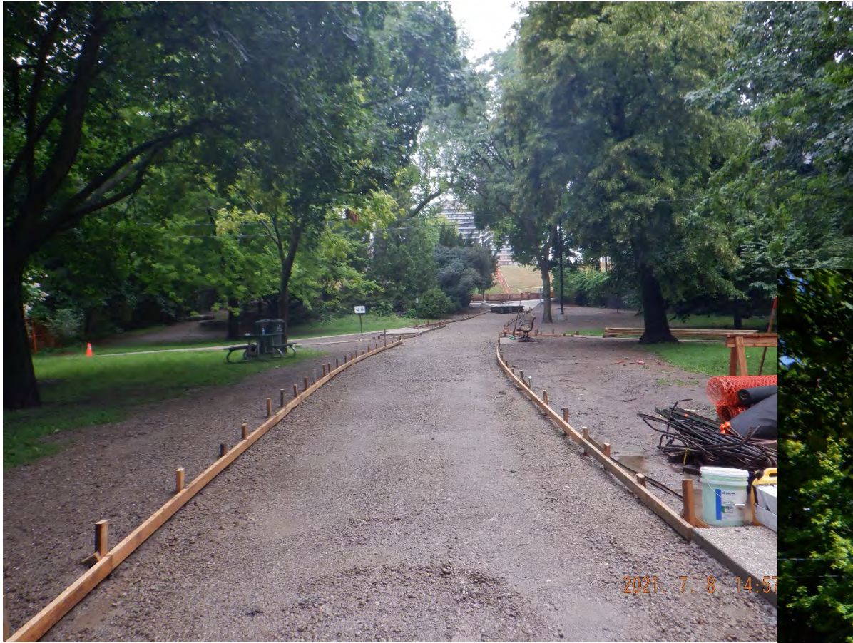
Little park driveway – forms & new concrete Looking north from Summerhill Avenue
