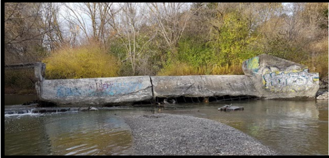
Photo of weir to be removed
