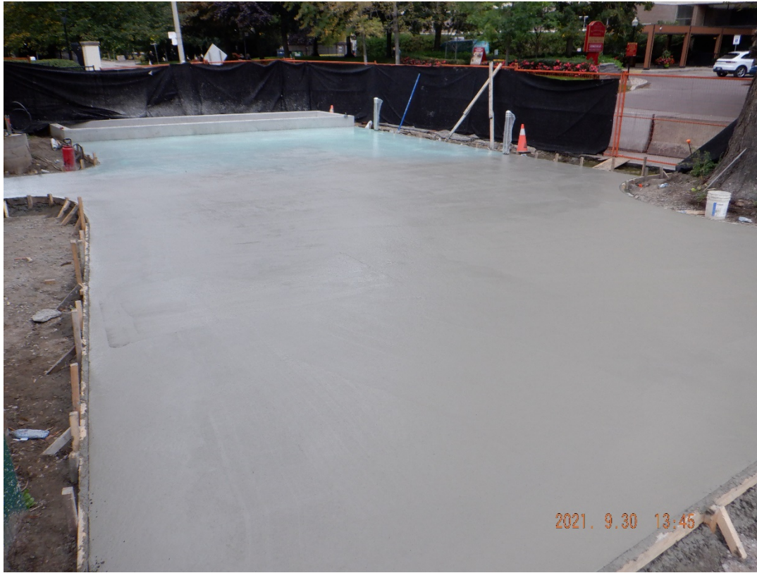
North-west corner of the park (Rosehill node) concrete poured and finished.
