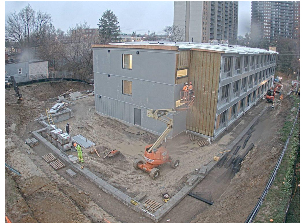
Construction of modular home at 11 Macey Ave.
