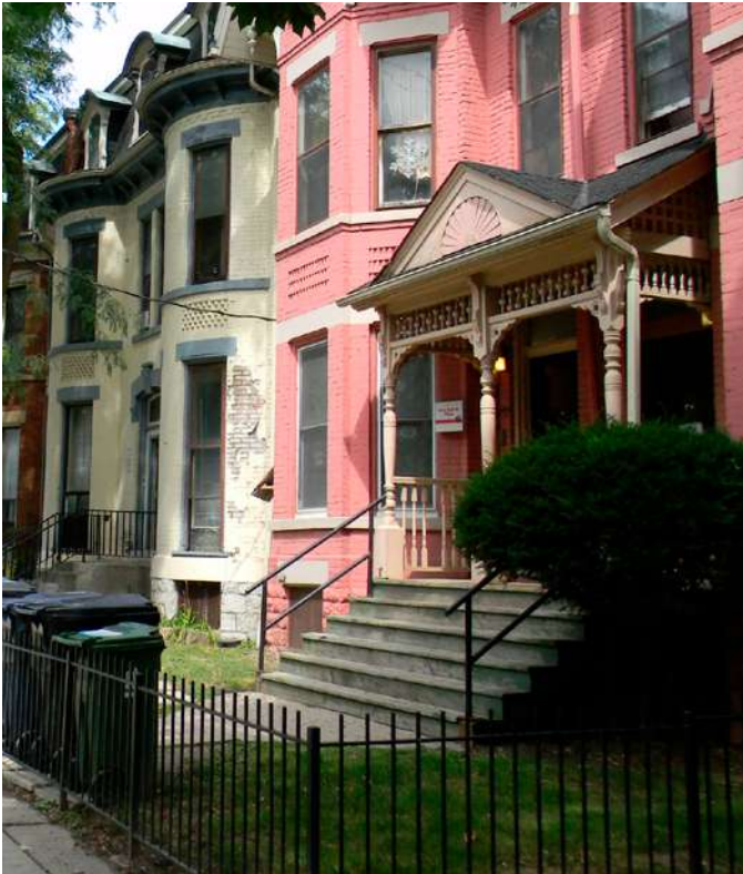
Figure 17: Entrance features of a contributing property in the Garden District HCD.
