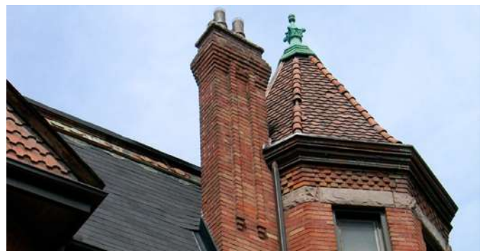
Figure 13: Turret roof in the Garden District HCD
