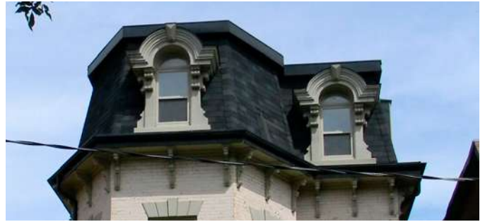
Figure 10: Mansard roof in the Garden District HCD
