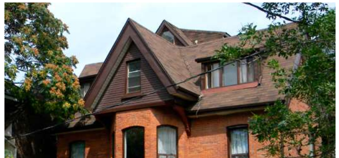
Figure 11: Gabled roof in the Garden District HCD
