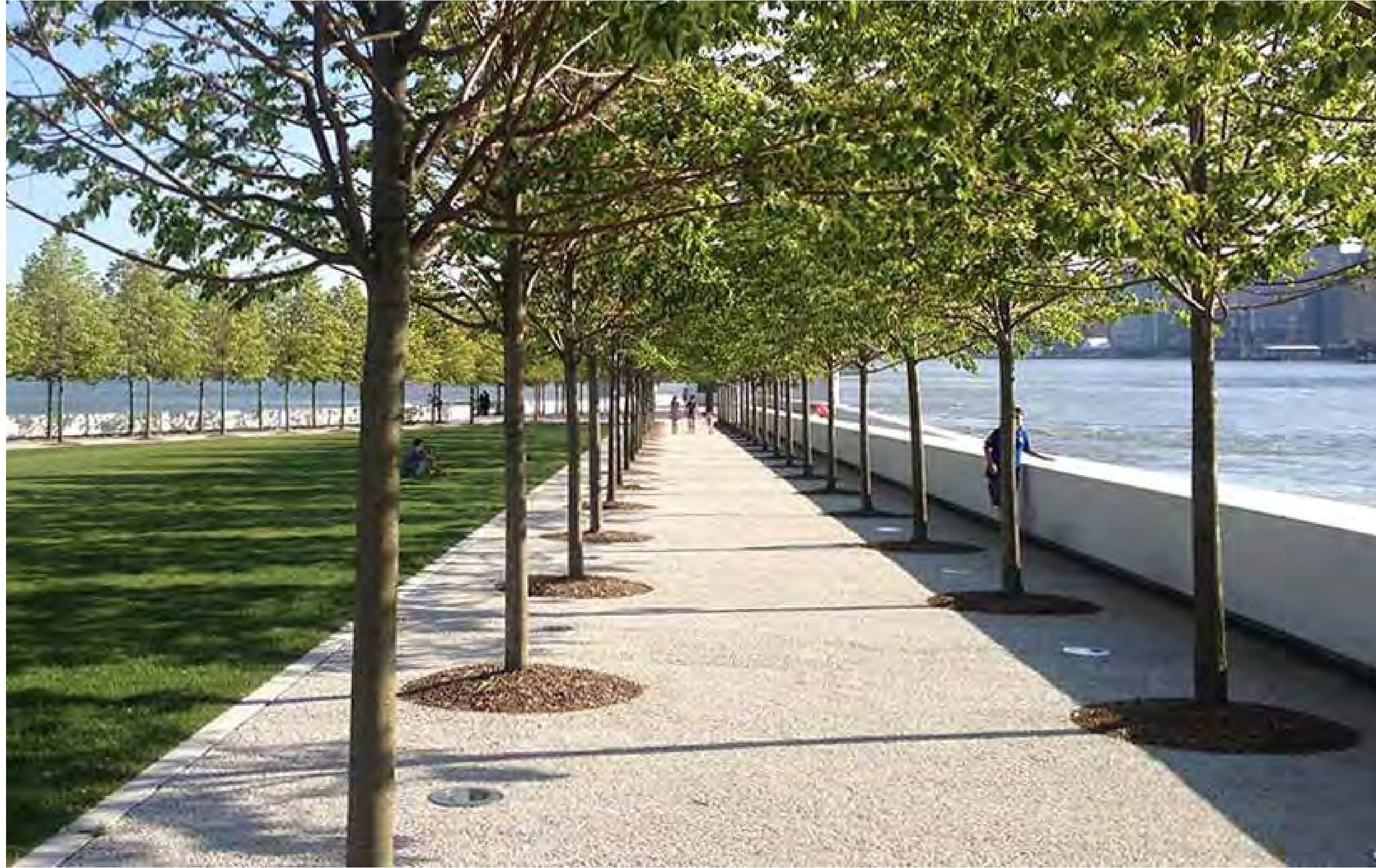
Permeable bonded granular paving in Four Freedoms Park in New York City
