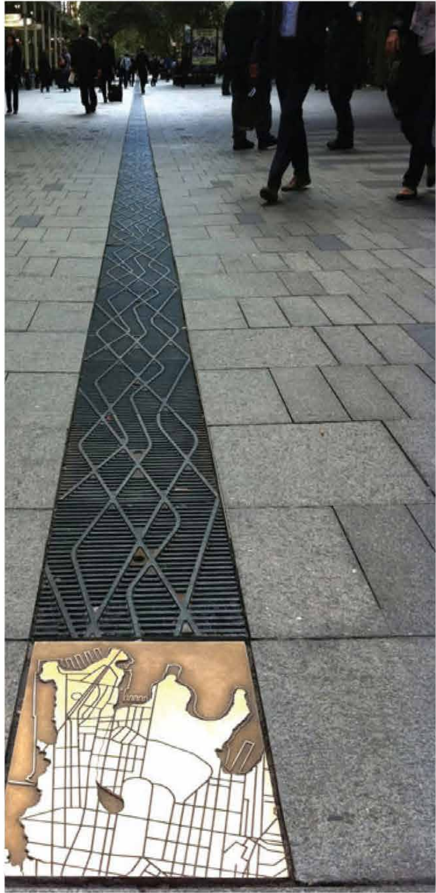
Runnels or drains capturing storm water and directing towards trees.
